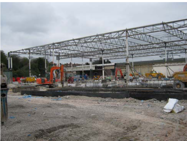
DP 5. E part of the site. View SW.
