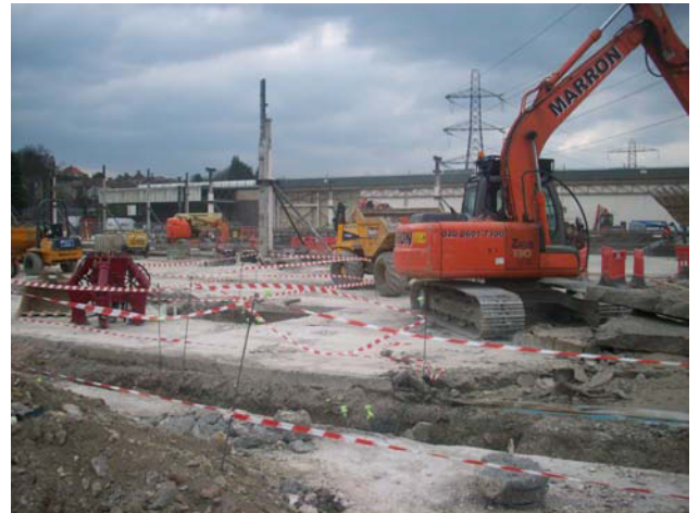
DP 2. E part of the site. View SW.
