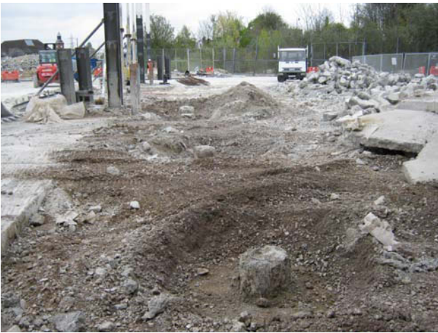
DP 9. S part of the site. View NE.
