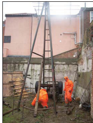
DP 4. Borehole Operation. View N
