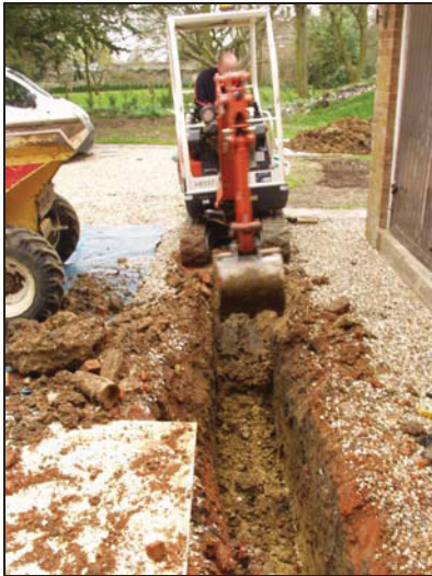
3 Foundation trench, W side of N extension. Looking N.
