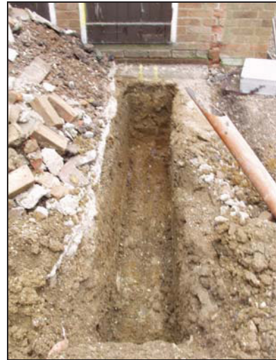
4 Foundation trench, E side of N extension. Looking N.
