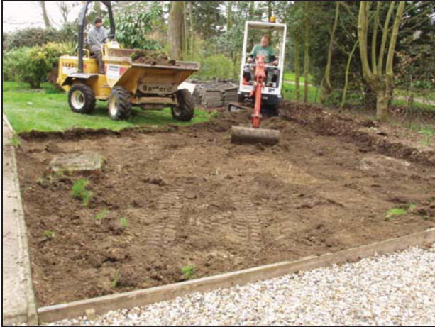
1 Footprint of cart lodge. Looking SW.
