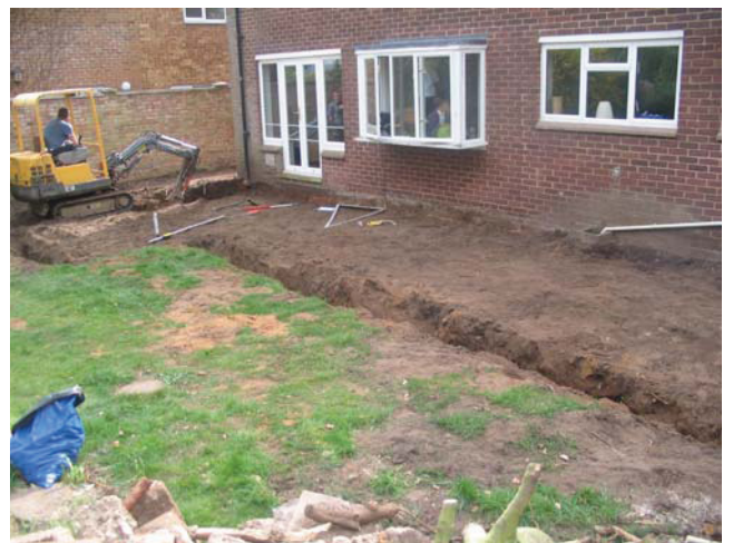
6 Excavated foundations. Looking south west.
