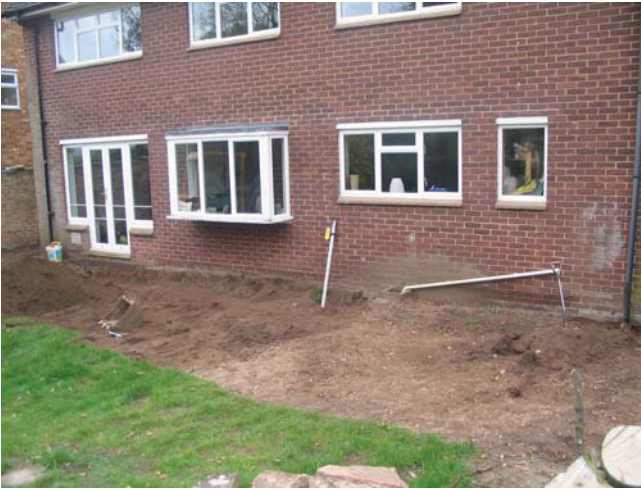
1 Footprint of house extension stripped of paving stones. Looking north east.
