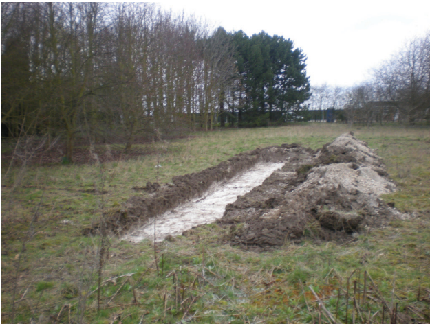
DP 13. Trench 3. View NW.
