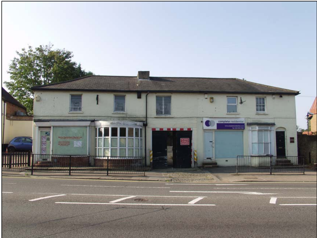
Plate 1 North elevation of the assessment buildings, taken from north (DP 02)
