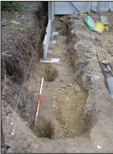
32 Fence foundation trench. Looking SE
