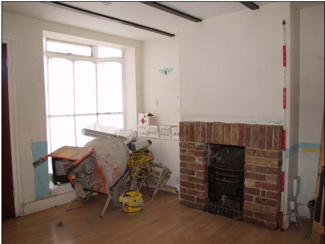
Plate 4 East side of Room 1 (No. 191), taken from the south-west (DP 12)
