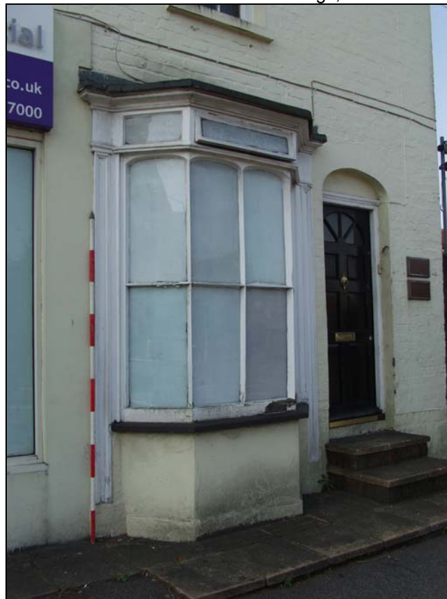
Plate 2 North elevation of No. 191 at ground floor level, taken from the north-east (DP 04)
