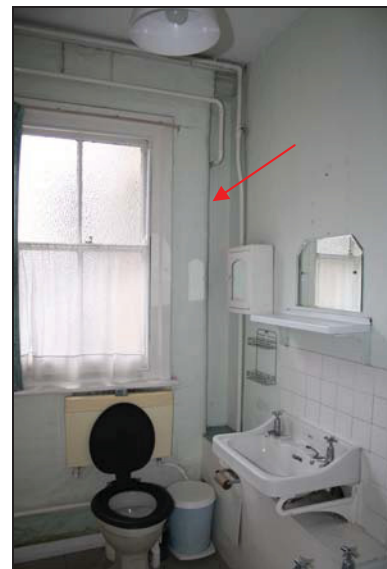
16 West side of the bathroom showing bevelled corner in brickwork (indicated), taken from the south-east
