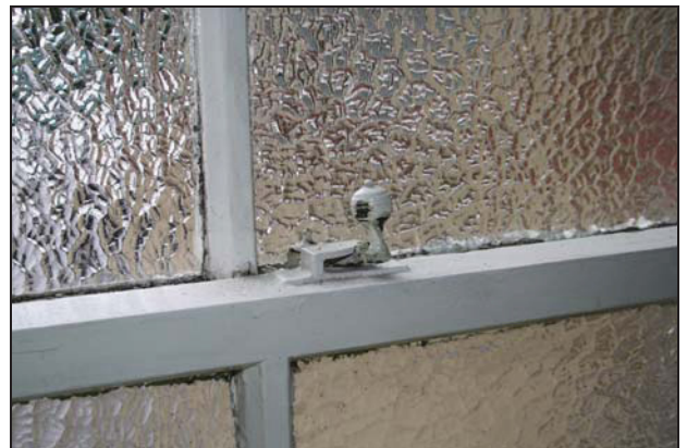
18 Sash catch on the window in the bathroom (Building 1), taken from the south-east
