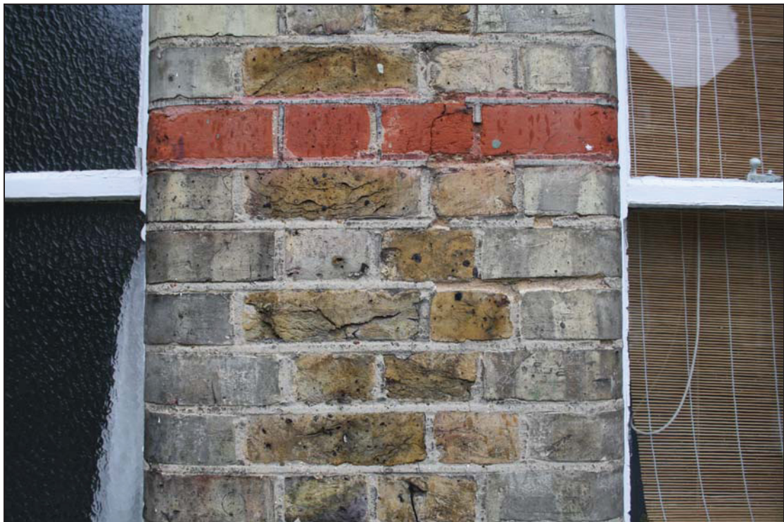
Plate 2 Sample of pilaster between windows on the west side of Building 1 showing bevelled corners to the jambs, taken from the west (DP 27)
