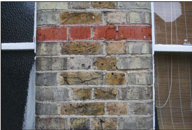
Sample of pilaster between windows on the west side of Building 1 showing bevelled corners to the jambs, taken from the west
