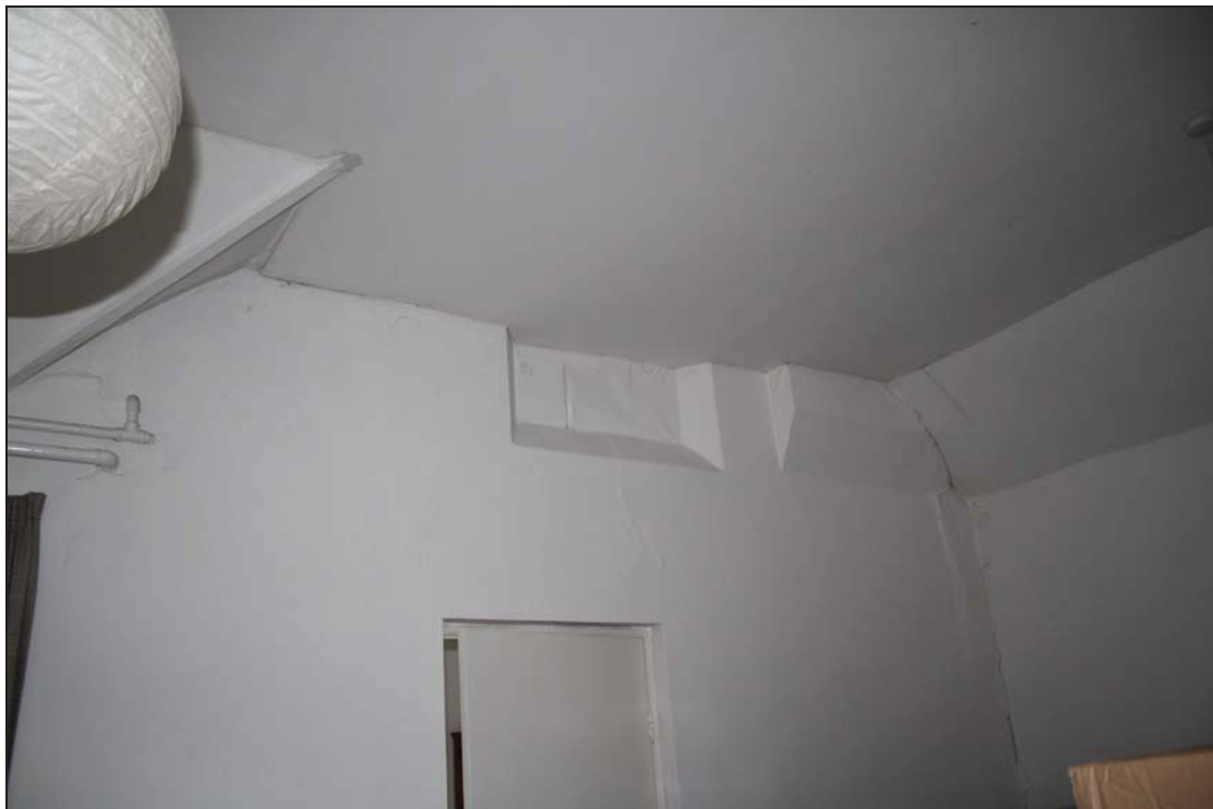
Plate 4 North wall of Room 1 (Building 1) showing high-level blocked aperture, taken from the south-west (DP 17)
