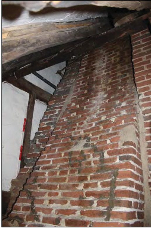
Plate 18 Chimney stack (Room 15), taken from the north-east (DP 45)
