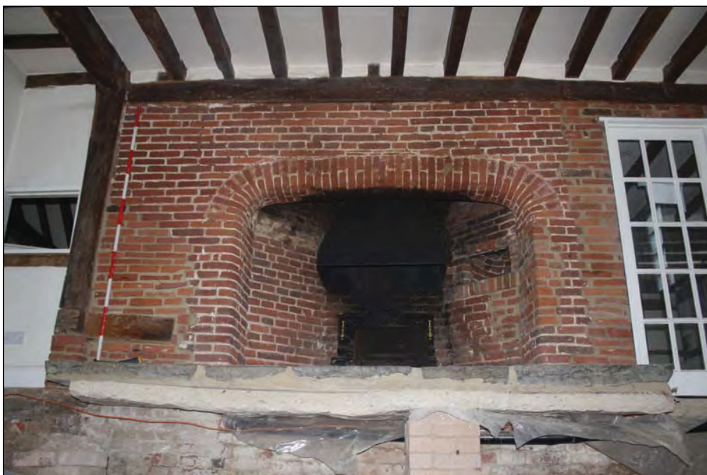
Plate 15 Fireplace (Room 5), taken from the north-west (DP 26)
