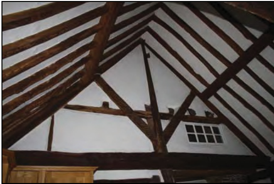
King post roof truss and original roof line, kitchen (Room 7), taken from the north-east
