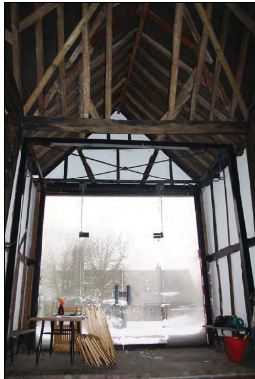
Plate 23 Midstrey showing modern alterations, taken from the south-west (DP 74)
