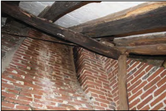
Soot blackened roof timbers (Room 15), taken from the north
