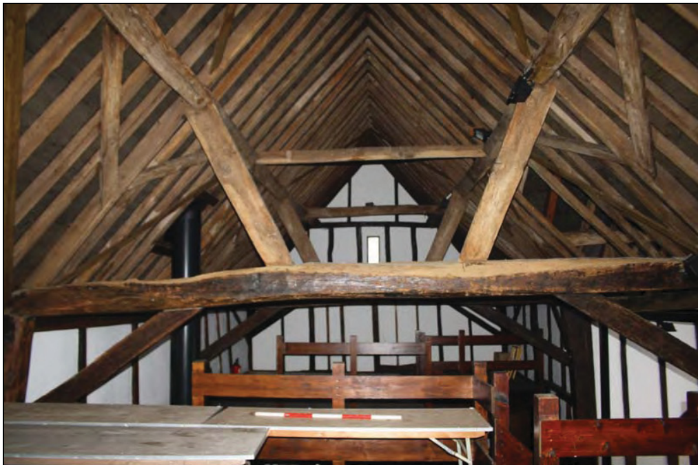
Plate 21 Roof construction, taken from the south-east (DP 78)
