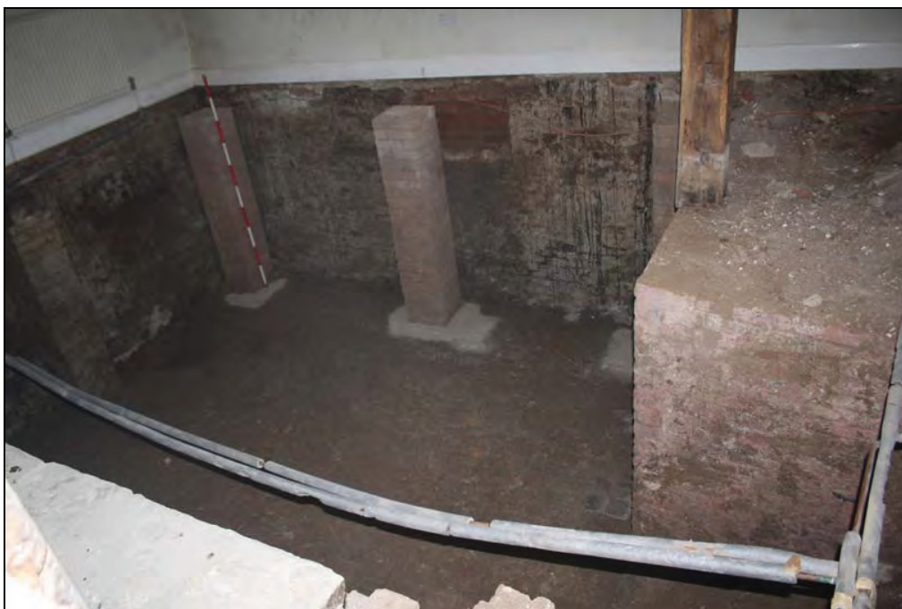
Plate 14 Cellar (Room 5), taken from the north-east (DP 28)
