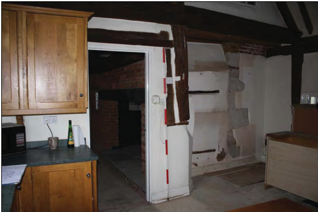
Plate 11 Kitchen (Room 7), taken from the north-east (DP 24)
