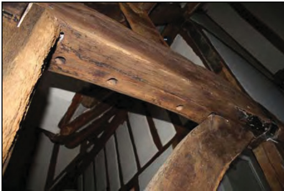
Assembly marks at principal bay division, first floor, taken from the north
