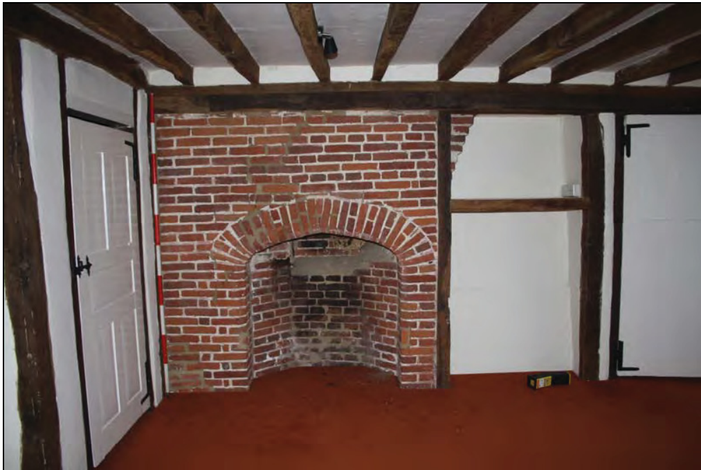
Plate 19 Fireplace (Room 16), taken from the north-west (DP 51)
