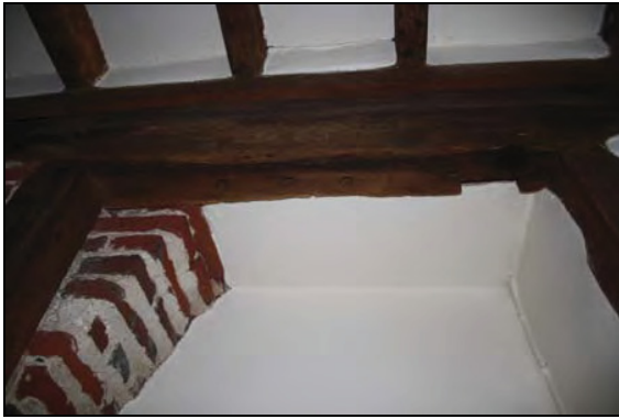
Panel groove (Room 17), taken from the west
