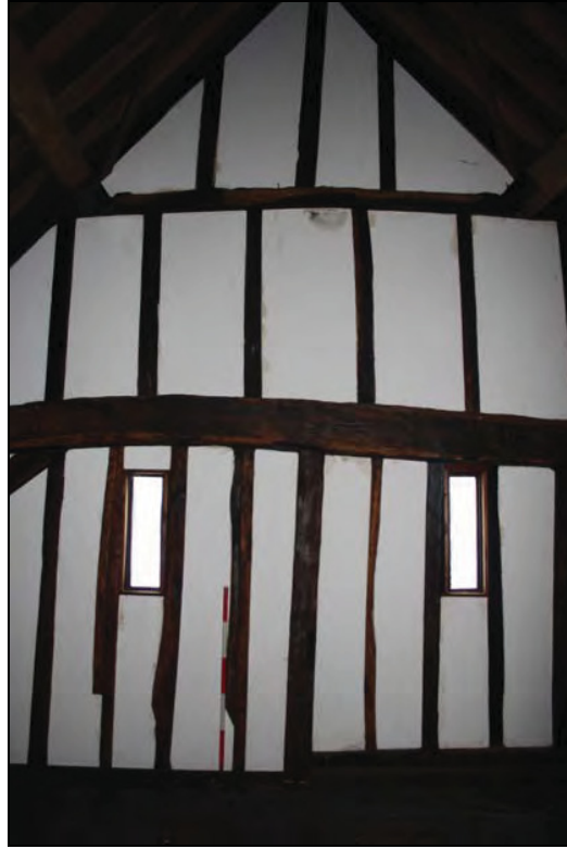
Plate 22 Northern truss, studs and wall panelling, taken from the north-west (DP 76)
