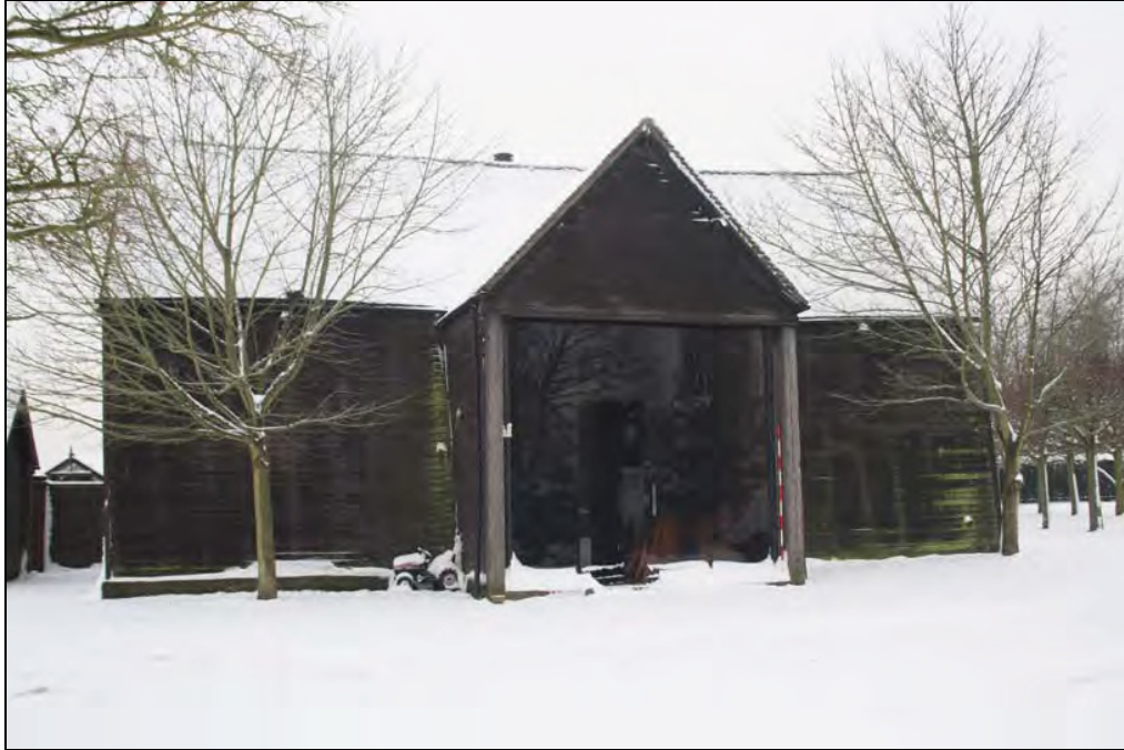
Plate 20 Barn, north-east elevation, taken from the north-east (DP 67)
