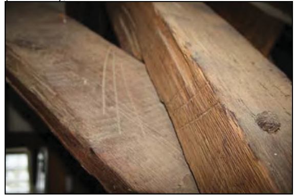
Empty mortise for wind brace with assembly marks (Room 14), taken from the south
