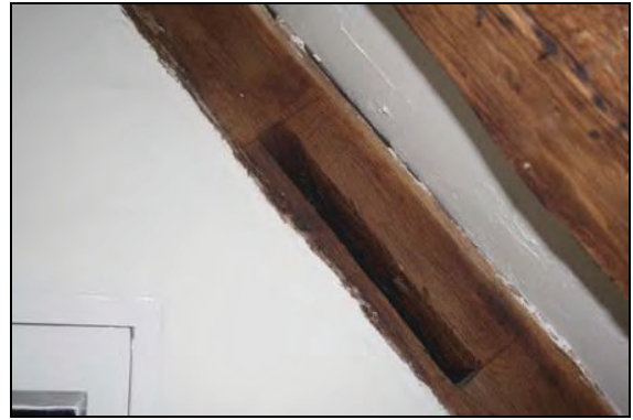
Empty mortise for wind brace with assembly marks (Room 14), taken from the south
