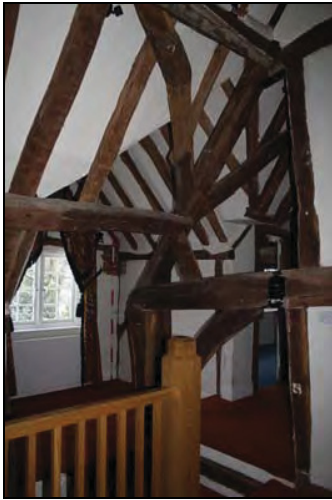
Alterations to the original structure to incorporate new staircase (Room 11), taken from the east
