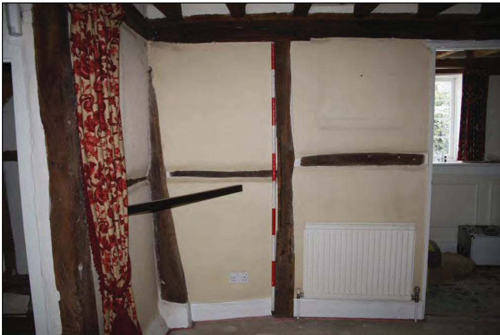
Plate 7 Living room (Room 6), ground floor, taken from the north-east (DP 20)
