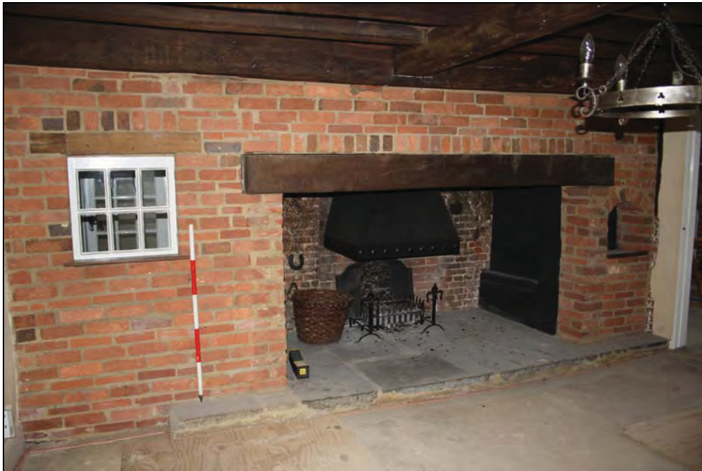
Plate 5 Inglenook fireplace, living room (Room 6), ground floor, taken from the south-East (DP 17)
