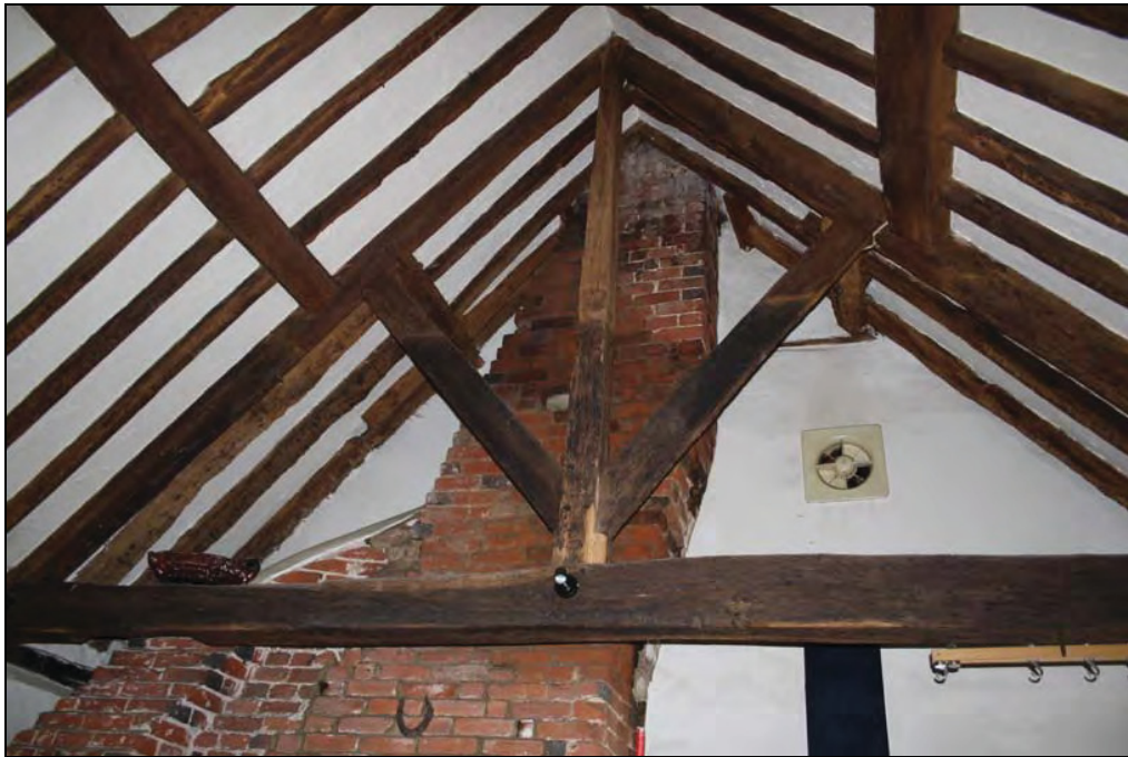
Plate 13 King post roof truss, kitchen (Room 7), taken from the south (DP 22)
