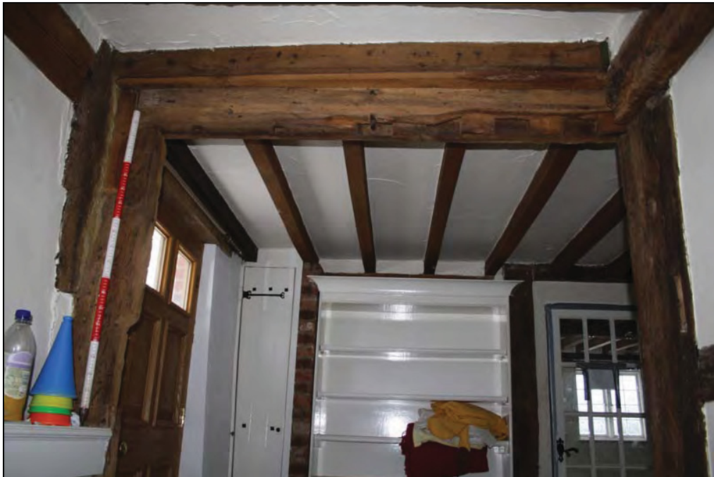
Plate 4 Lobby entrance (Room 1), taken from the south-east (DP 13)
