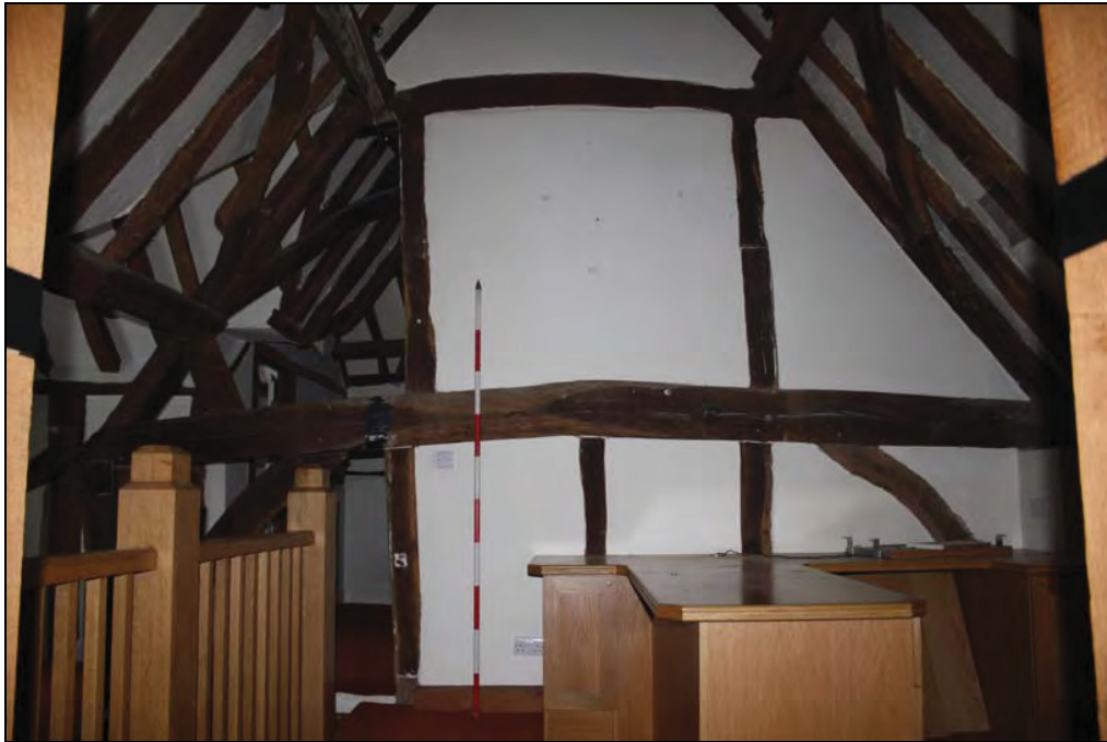
Plate 16 Queen post roof truss (Room 10), taken from the south-east (DP 36)
