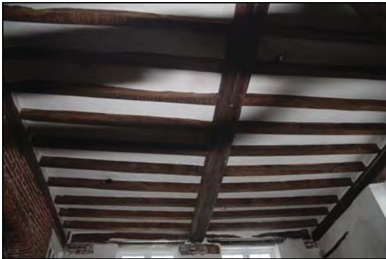
King post roof truss and original roof line, kitchen (Room 7), taken from the north-east
