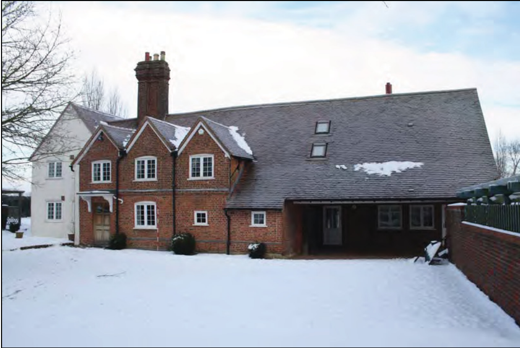
Plate 1 Gyfres Farm, south-west elevation taken from the south (DP 1)
