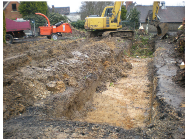
DP 6. Trench 3. View SSW.
