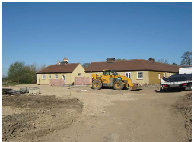
DP 4. S part of the site. April 2010. View N.
