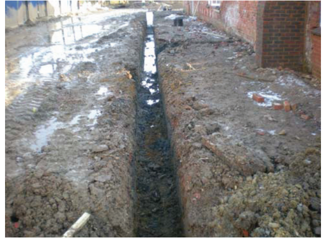
DP 14. Service trench to the E of 'stock' buildings. View SE.
