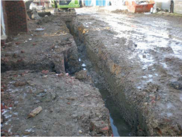
DP 13. Service trench to the E of 'stock' buildings. View NNW.
