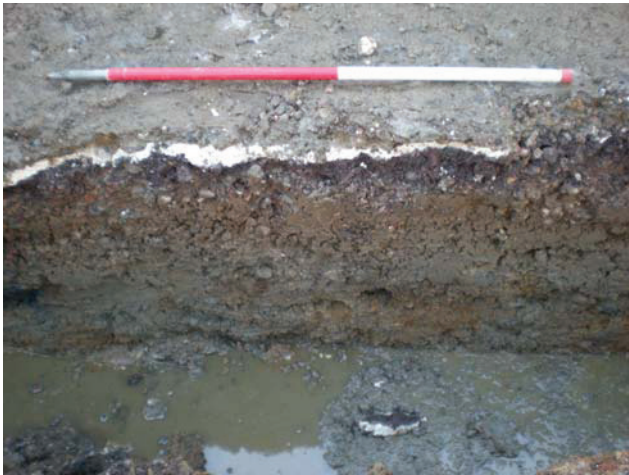
DP 15. Service trench to the E of 'stock' buildings. Sample section 3. View NE.
