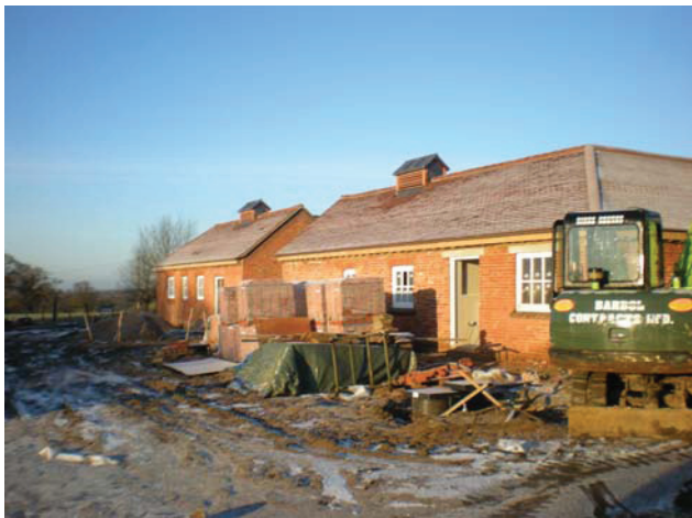
DP 3. S part of the site. February 2010. View NW.
