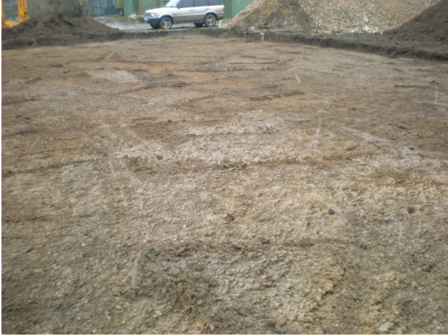
DP 7. W part of the S barn area. View S.
