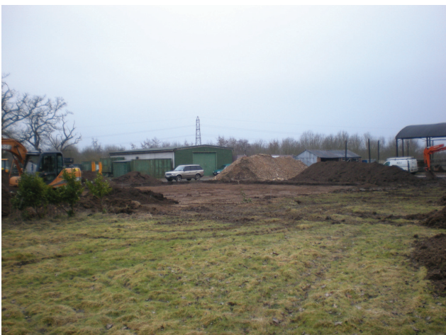
DP 5. Area of the proposed S barn. View S.
