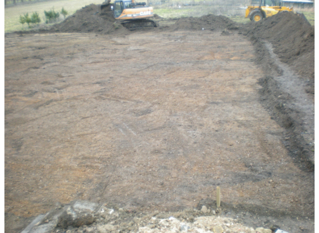
DP 8. S part of the S barn area. View NE.
