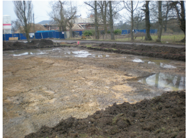
DP 4. N part of the N barn area. View N.
