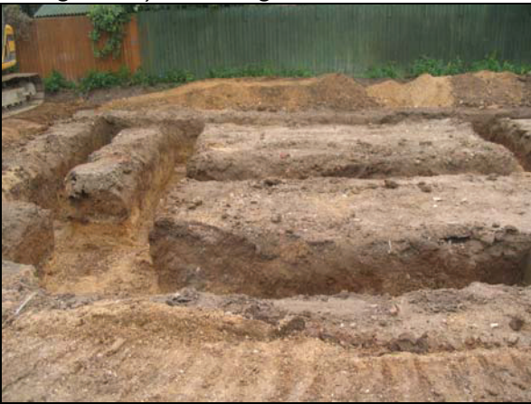
3 Foundation trenches of house. Looking NE
