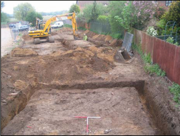
1 Footprint of garage (foreground) and house (background). Looking NE.
