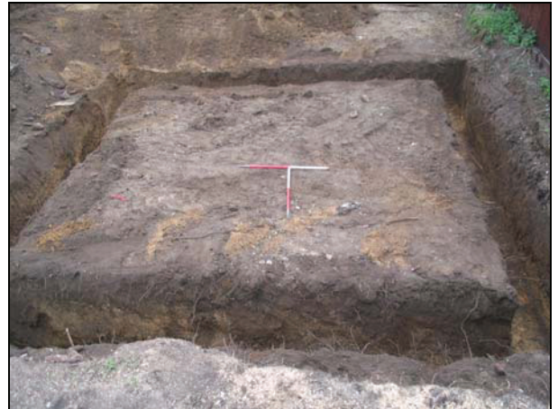
2 Foundation trench of garage. Looking NE.
