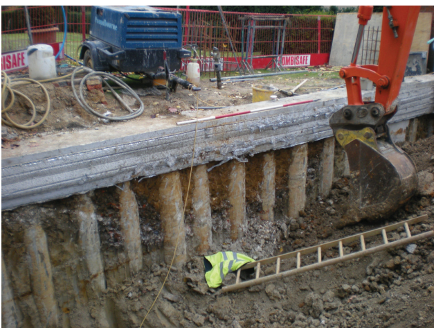
DP 5. SE side of the excavation with F1004. View S.
