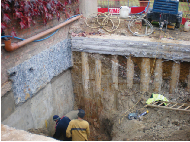
DP 7. E corner of the excavation. View ESE.
