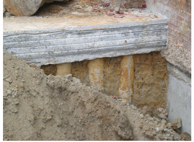
DP 8. W corner of the excavation. View W.
