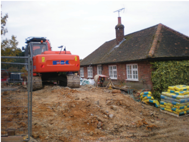
DP 3. Excavation area. View S.
