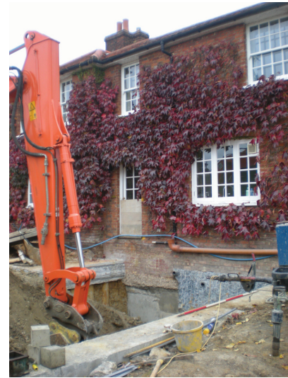
DP 2. The groundworks. View N.
