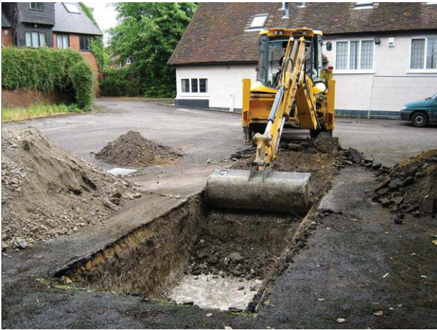
DP 7 Excavation of Trench 2. View NNE
