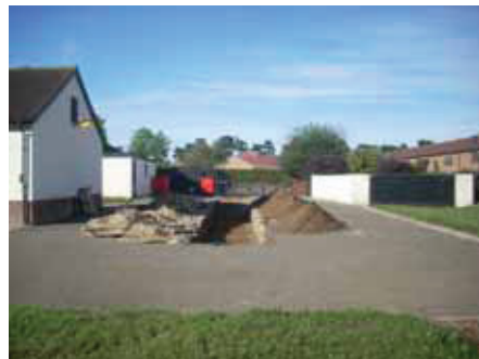
DP 6. Site. View NW
