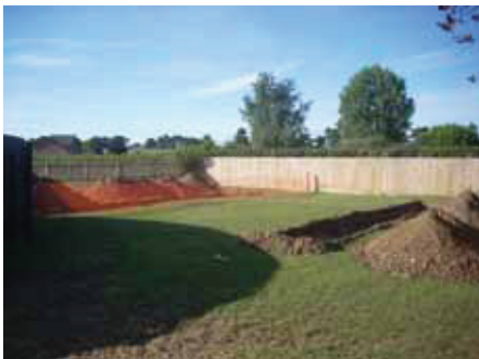
DP 5. Site. View S
