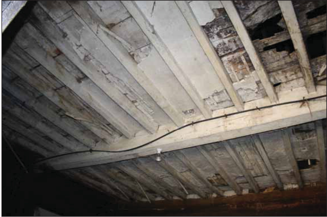
Plate 9 Building 4, interior, ground floor ceiling, taken from the north-west (DP 26)
