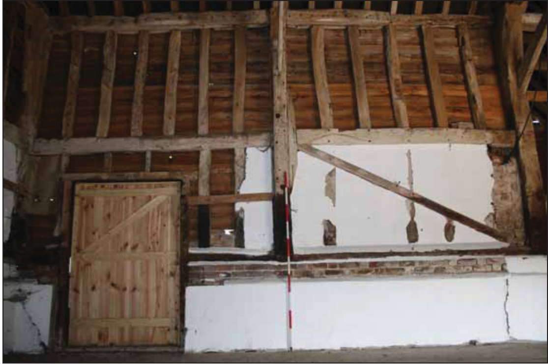
Plate 3 Building 1, interior, northern elevation, bays 4 & 5, taken from the south (DP 12)
