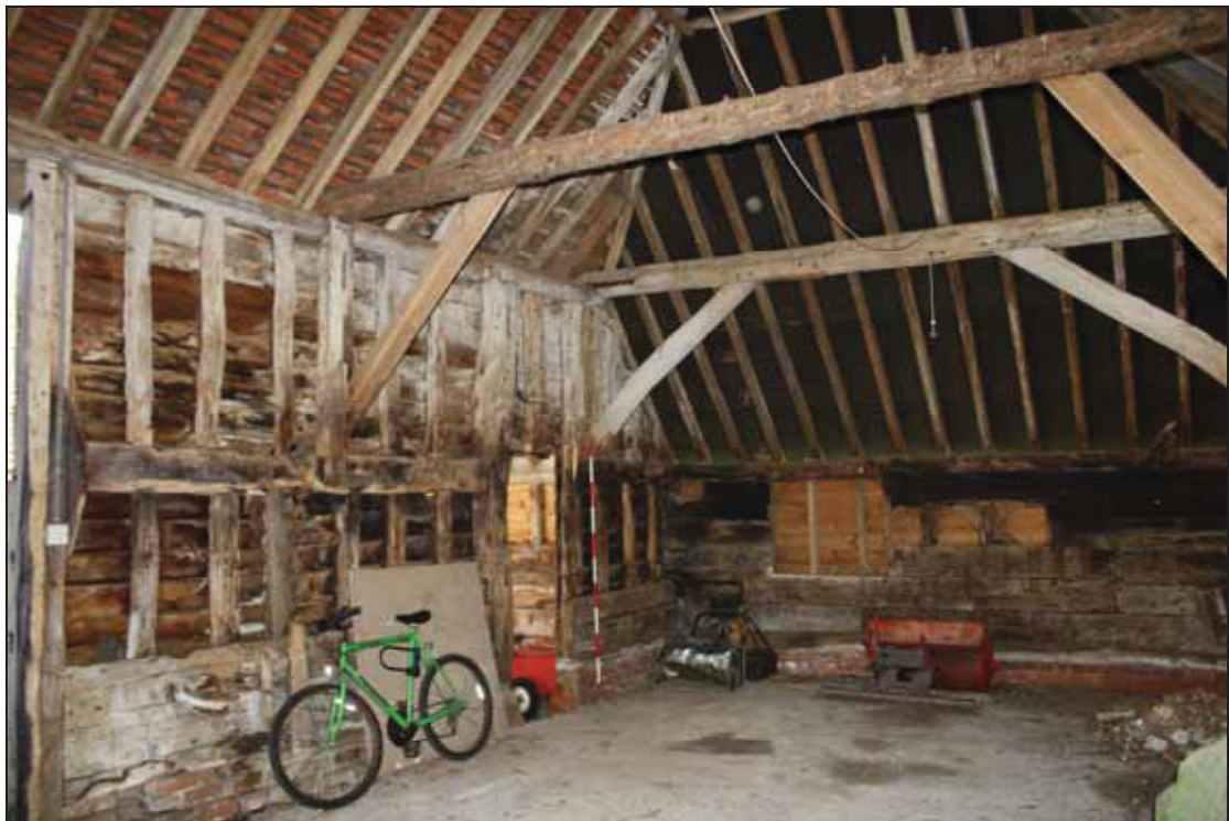
Plate 8 Building 3, interior, taken from the south-west (DP 24)
