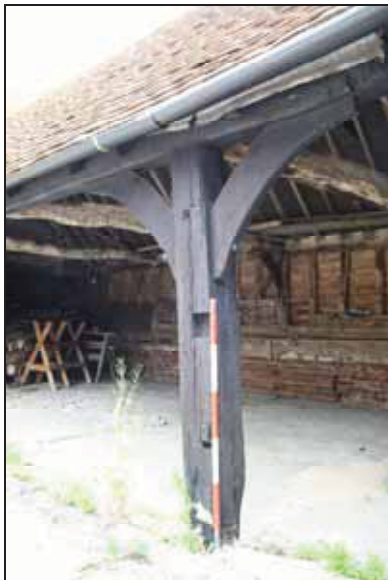
Building 2, braced post at open bay division, taken from the south-west
