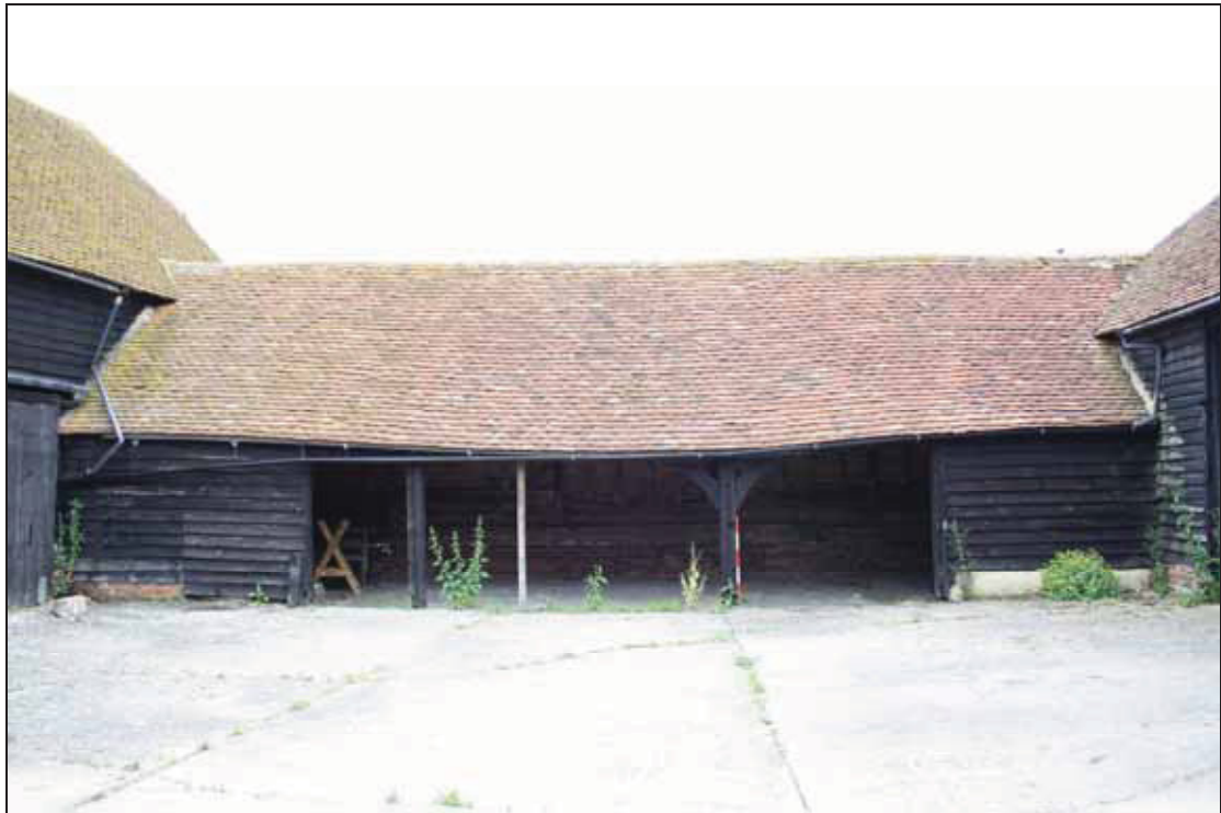
Plate 5 Building 2, western elevation, taken from the west (DP 45)
