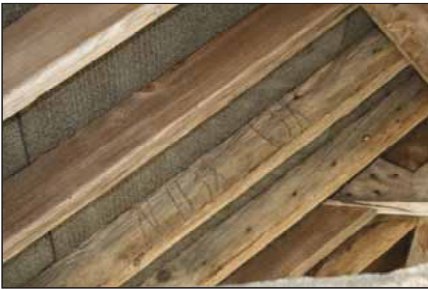
Building 4, interior, chamfered bridging joist with lamb's tongue stops, taken from the north-east
