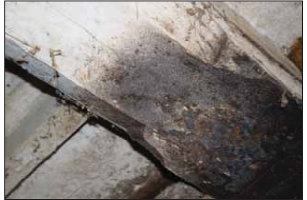
Building 1, interior, principal post of truss 4 displaying assembly mark 'IV', taken from the north-east
