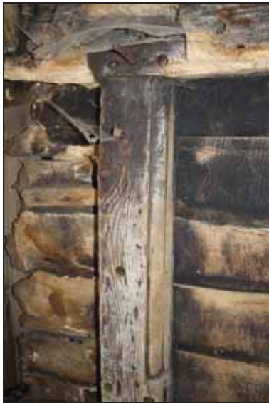
Building 3, interior, window moulding on piece of re-used timber, taken from the south
