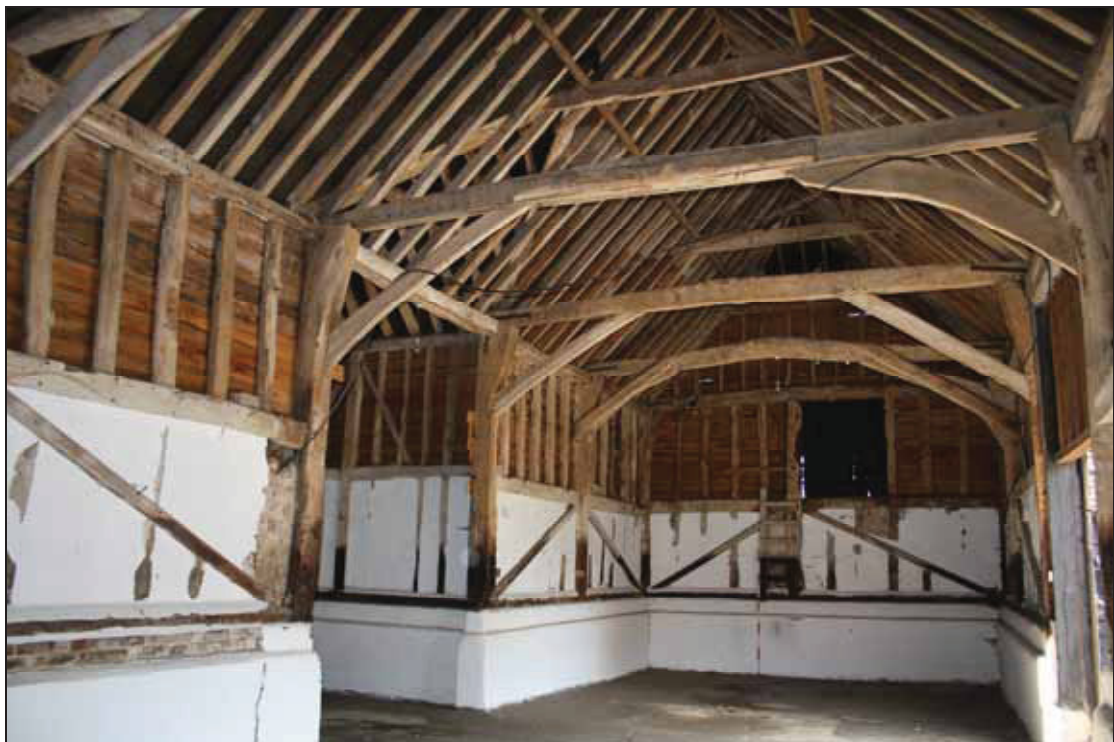
Plate 2 Building 1, interior, taken from the south-west (DP 5)
