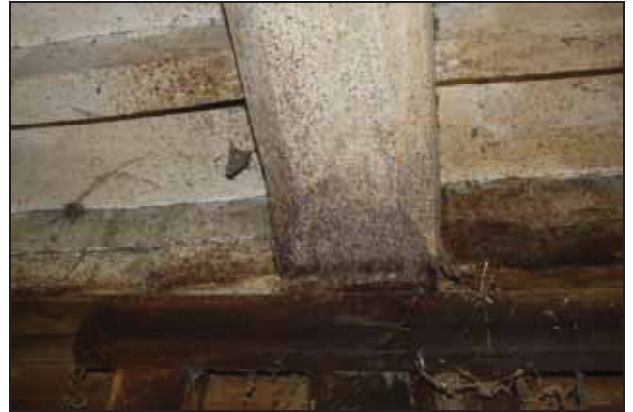
Building 4, interior, chamfered bridging joist with lambs tongue stops, taken from the north-east
