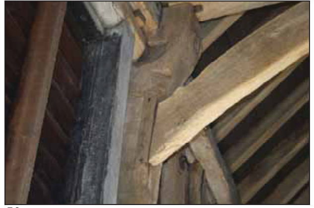
Building 1, interior, principal post of truss 4 displaying assembly mark 'IV', taken from the north-east
