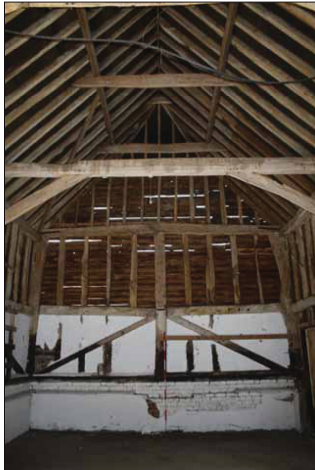
Plate 4 Building 1, interior, truss 6, western elevation, taken from the east (DP 16)
