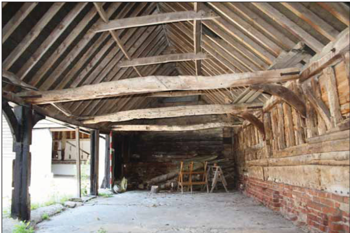
Plate 6 Building 2, interior, taken from the south (DP 18)
