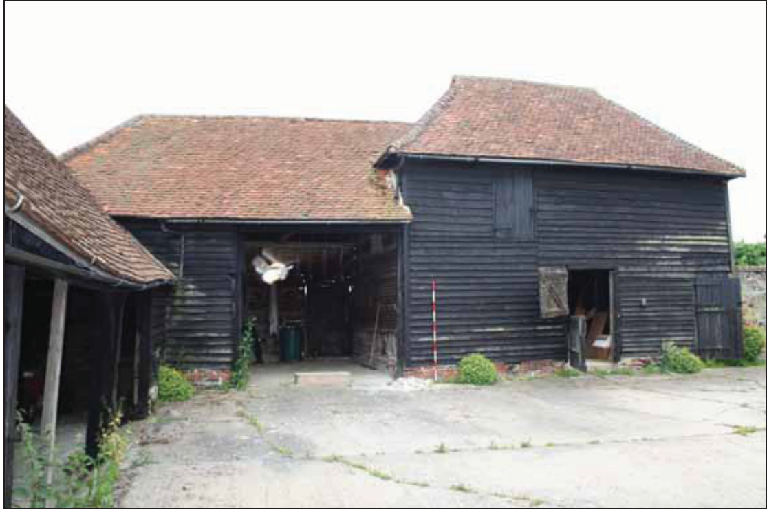
Plate 7 Buildings 3 & 4, northern elevations, taken from the north-east (DP 46)
