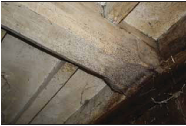
Building 4, interior, chamfered bridging joist with lamb's tongue stops, taken from the north-east
