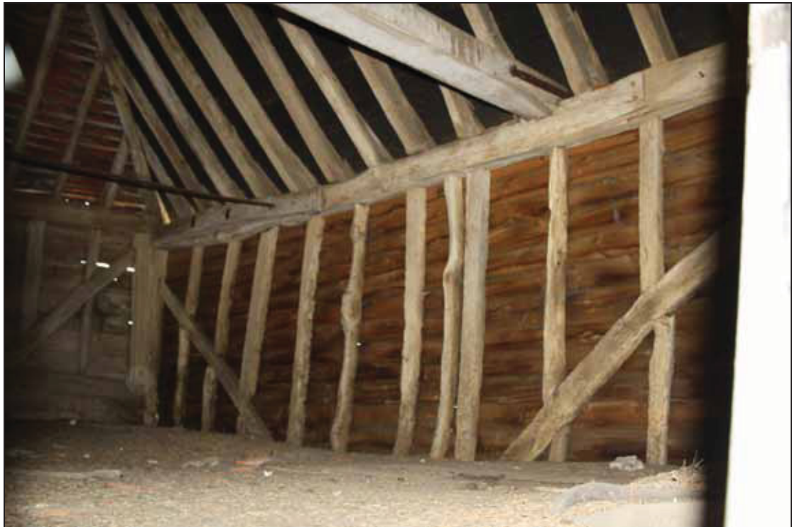
Plate 11 Building 4, interior, first floor, southern elevation, taken from the north-west (DP29)
