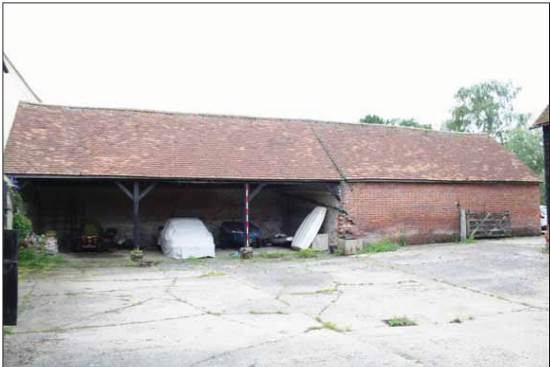
Plate 12 Building 5, eastern elevation, taken from the south-east (DP 48)
