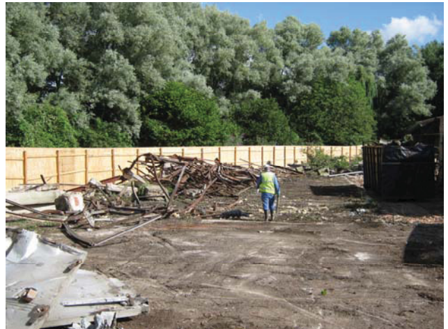
DP 2. N part of the site. View NE.
