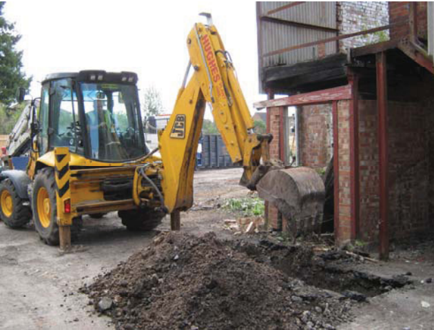
DP 3. Excavation of test pit. View SE.
