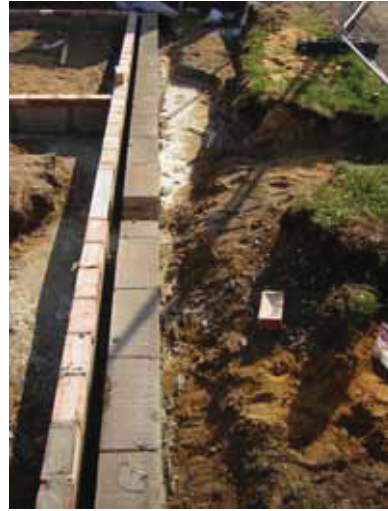
DP 2. Concrete footings, west facing
