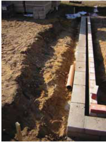
DP 1. Concrete footings, east facing
