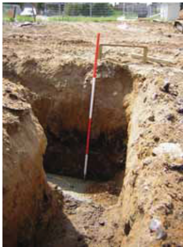
DP 4. Footing trench showing peat layer, east facing
