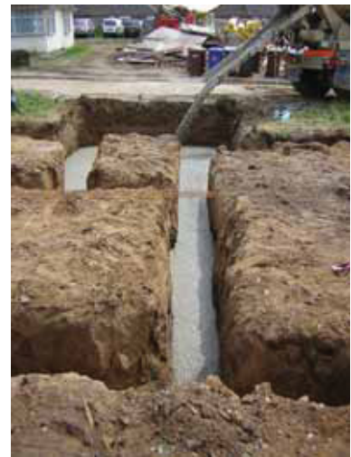
DP 4. Concreting footing trenches, east facing
