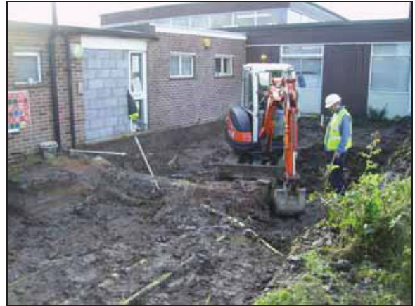
2 General view of the site, working shot. Looking south-west
