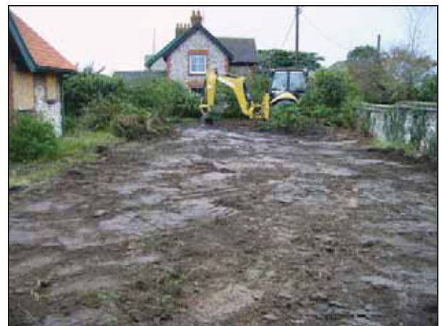
12 General view of the site
