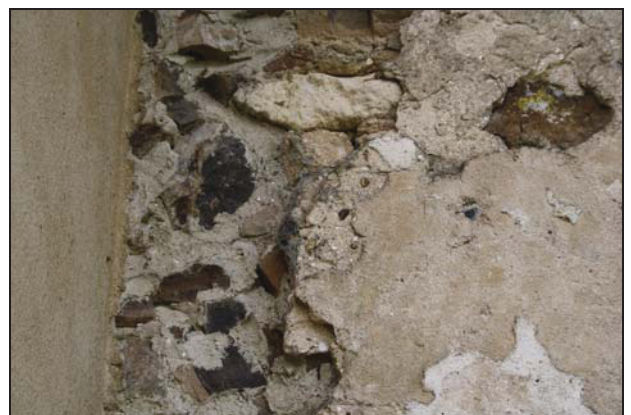
Possible putlog hole (P1) in Bay 3, north nave wall, taken from the north
