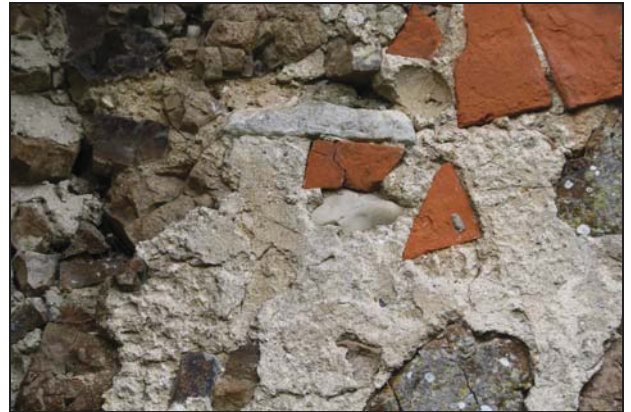
Possible putlog hole (P3) in Bay 1, north nave wall, taken from north
