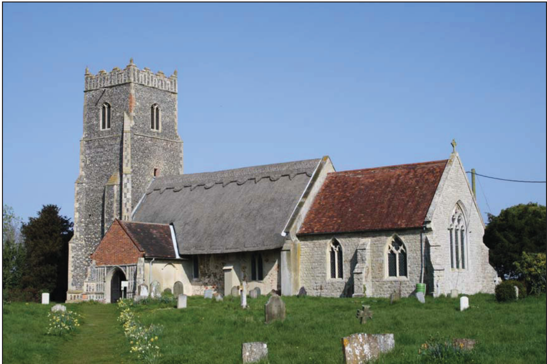
1 General view of the church, taken from the south-east (48)
