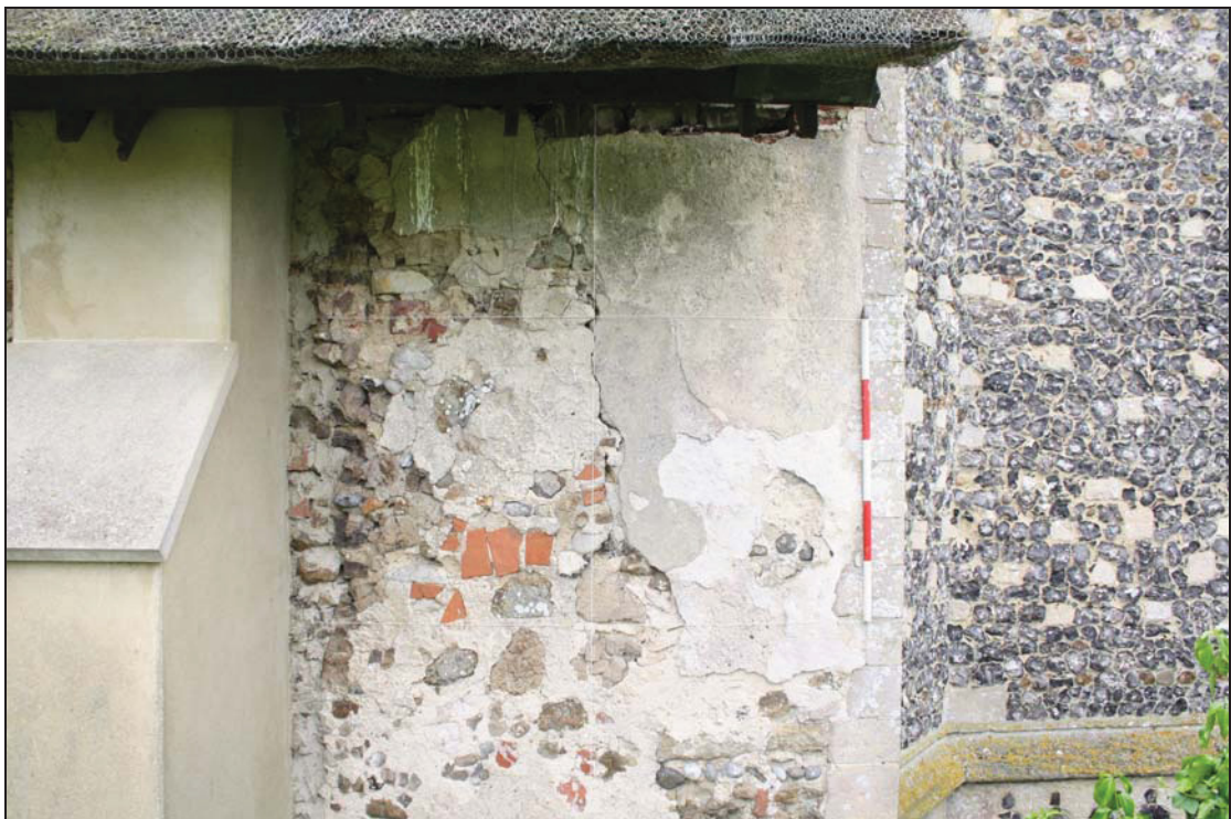
4 Detail of north nave wall, Bay 1, taken from the north (12)
