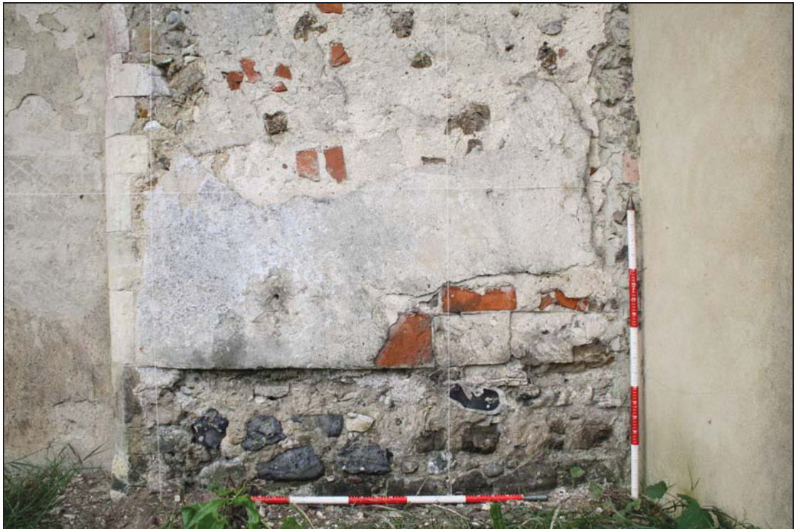
5 Detail of north nave wall, Bay 2, taken from the north (36)
