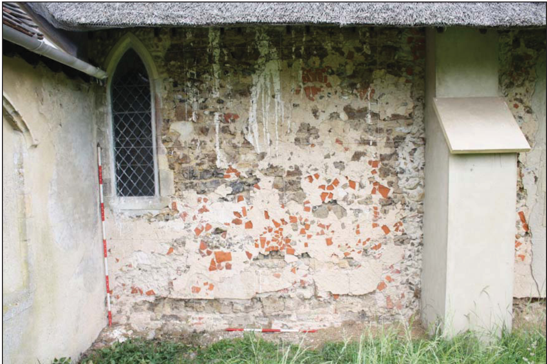
11 South nave wall, Bay 3, taken from the south (15)
