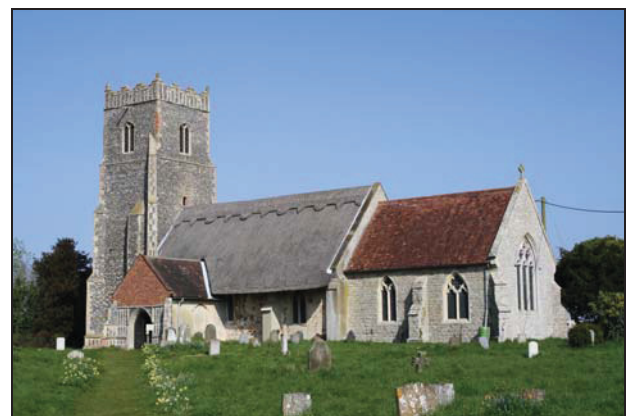
48 General view of the church, taken from the south-east
