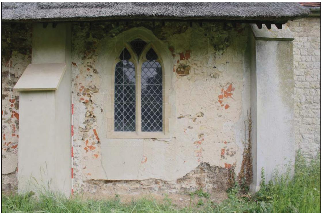
12 South nave wall, Bay 4, taken from the south (22)
