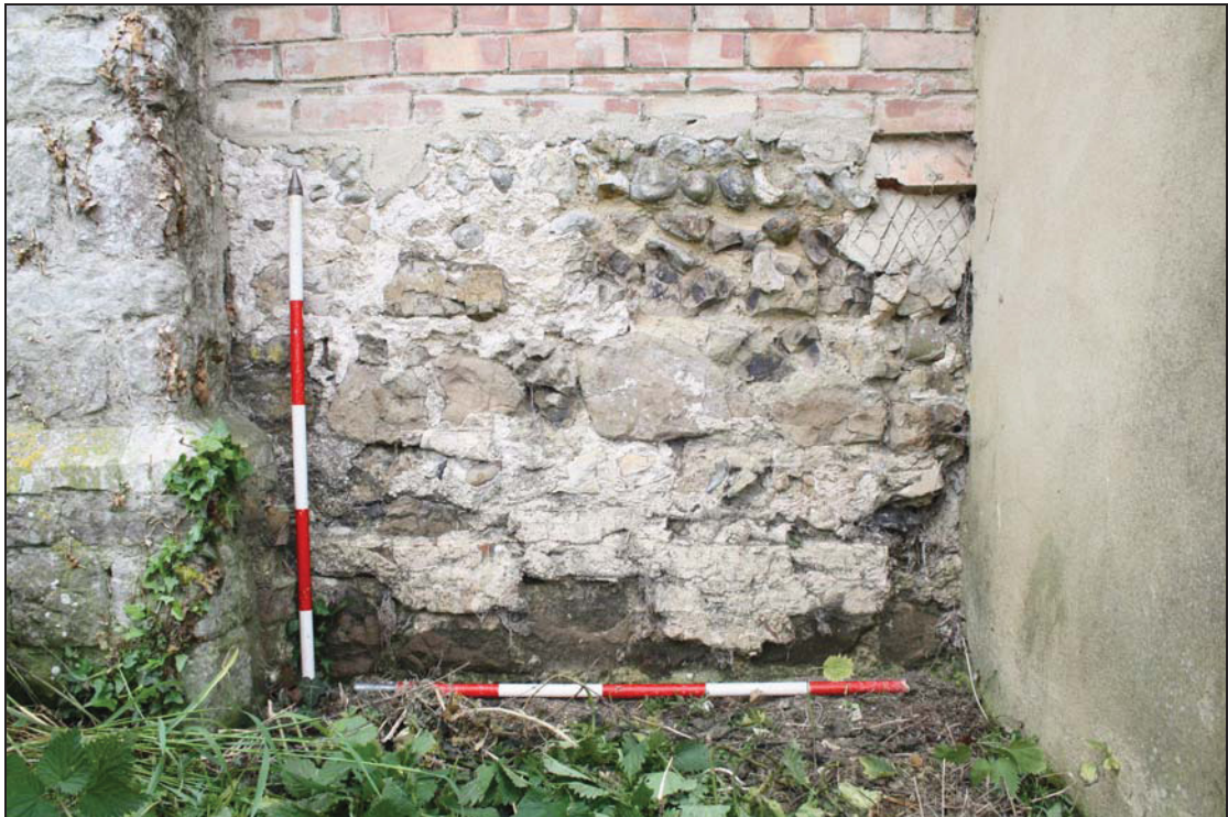
9 North nave wall, lower Bay 4, taken from north (01)
