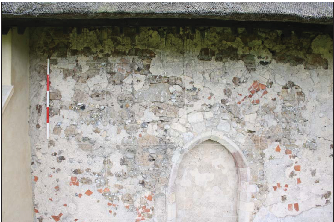
6 Detail of north nave wall, Bay 2, taken from the north (09)
