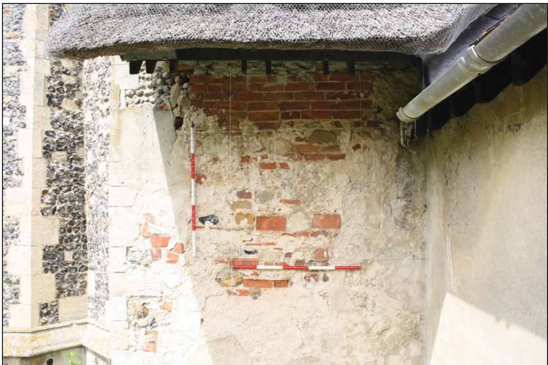
10 Detail of south nave wall, Bay 1, taken from the south (14)
