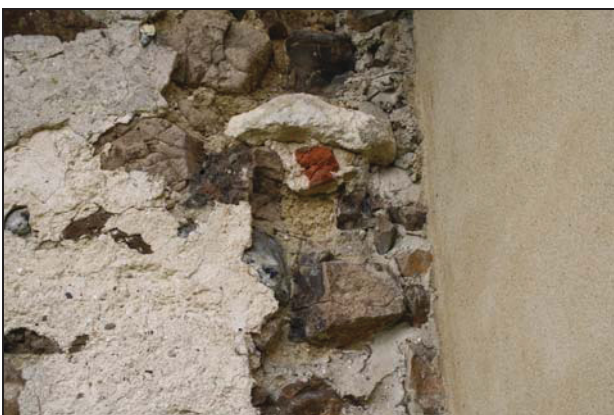
Putlog hole (P2) in Bay 3 north nave wall, taken from the north
