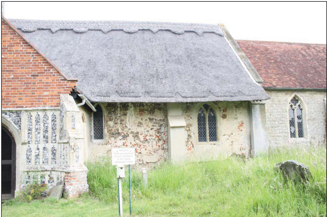
2 Detail of south nave wall, Bay 1, taken from the south (37)
