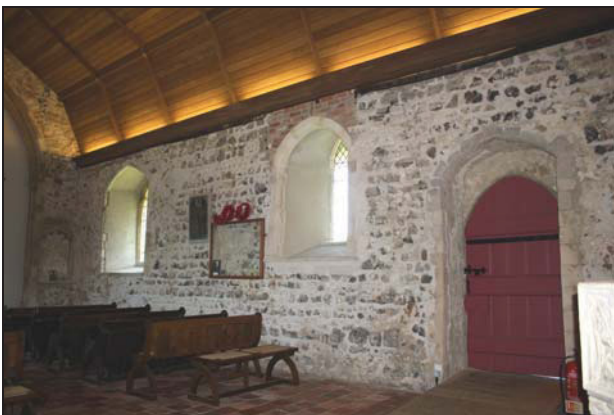
45 Internal façade of the south nave wall, taken from the north-west
