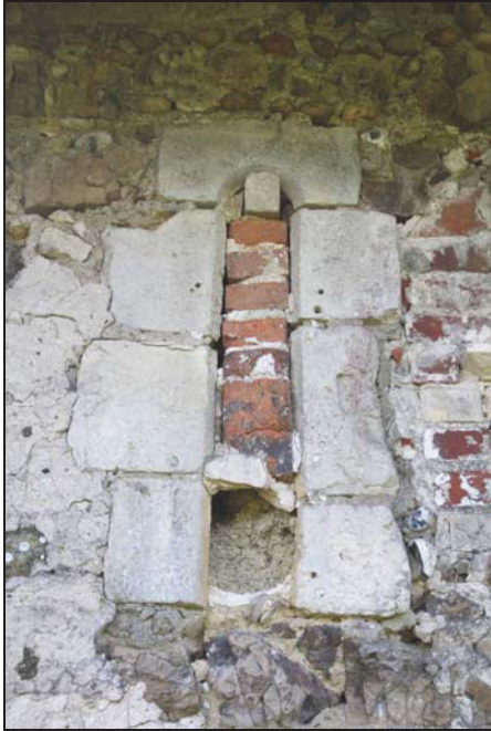
43 Detail of original lancet window in Bay 3, north nave wall, taken from the north
