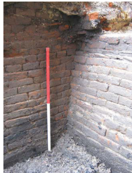
DP 10. NE corner of the basement. M1007 and M1004. View NNE.
