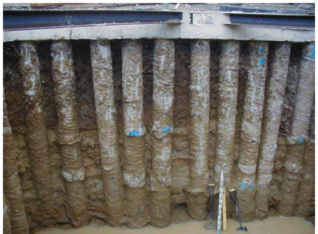
DP 6. S section of the excavation. View S.
