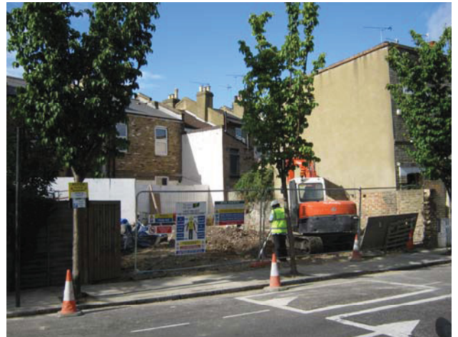
DP 2. Rear of No. 94 Glenthorne Road. View SW from Redmore Rd.
