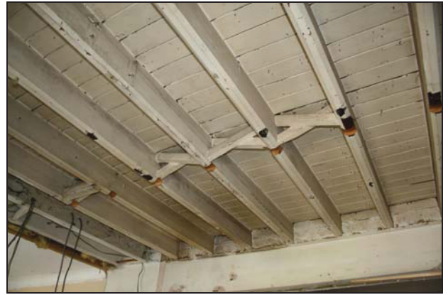
Detail of ceiling form showing laced bracing in Area 1 (Range 1, lower level), taken from the north
