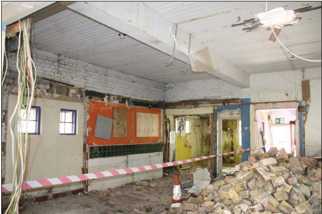
7 View of Area 3 (Range 1, lower level), taken from the north-west (27)
