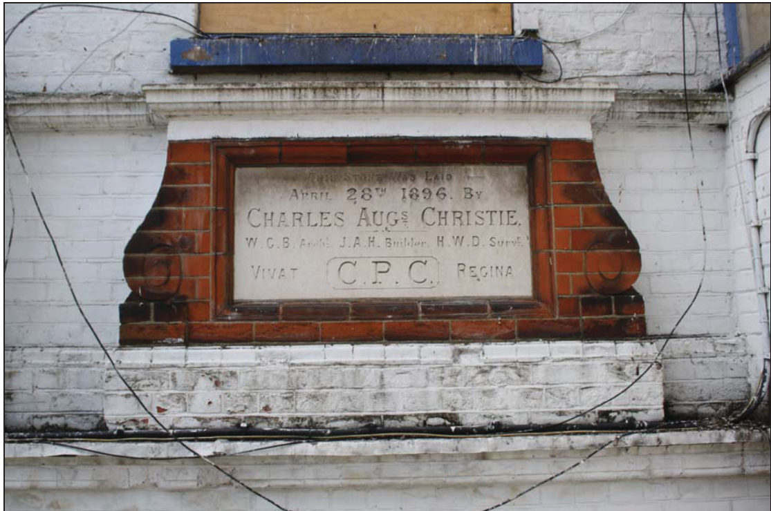
5 Foundation stone on the east side of Range 2 at upper level, taken from the east (06)
