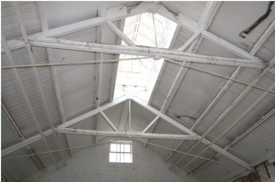
10 Roof structure of Range 2, taken from the east (17)
