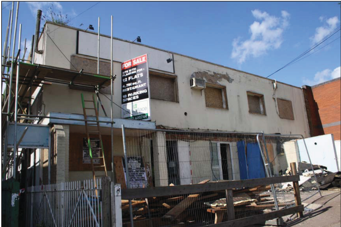
1 North façade of Range 1, taken from the north-east (04)
