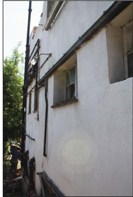
46 East façade of Range 1, taken from the north-east
