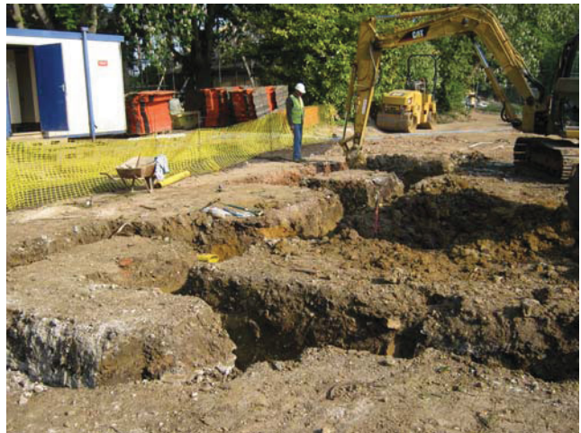
DP 16. Plot 6, excavation of foundation trenches. View NW.
