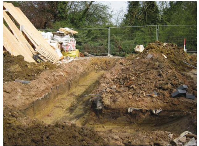
DP 2. Trench 1. View NNW
