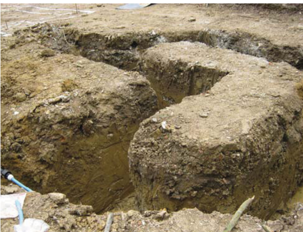
DP 17. Plot 6, SW foundation trenches. View SE.
