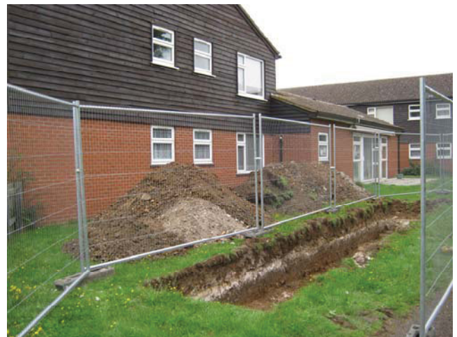
DP 6. S part of the site with Trench 2. View NE.
