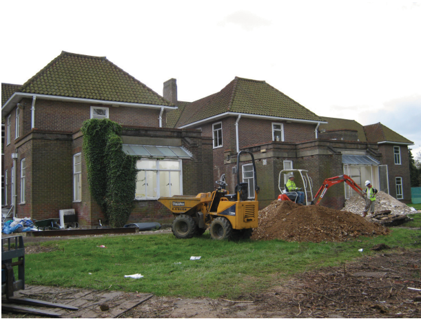
DP 1 General view of site, looking south
