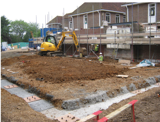
DP 5 View of site looking south
