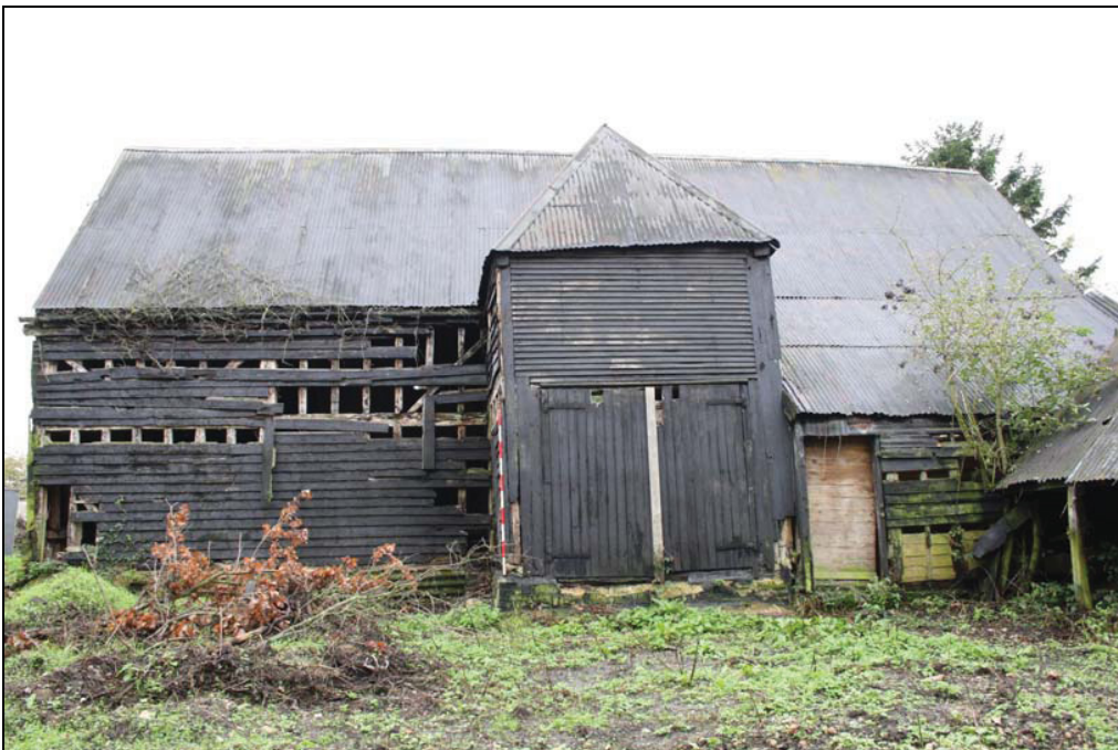
Plate 2 Barn, Tile Kiln Farm, north-eastern elevation, taken from the east (DP 4)
