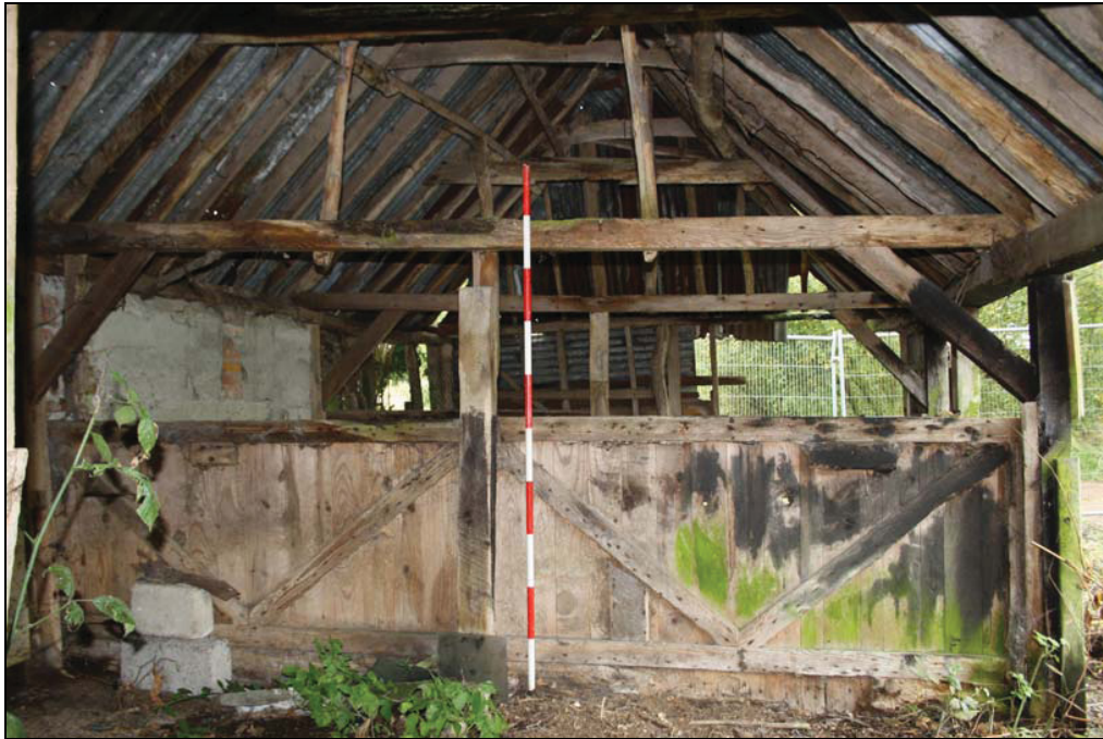
Plate 9 Stall partition, animal byre, interior, taken from the south-west (DP 11)
