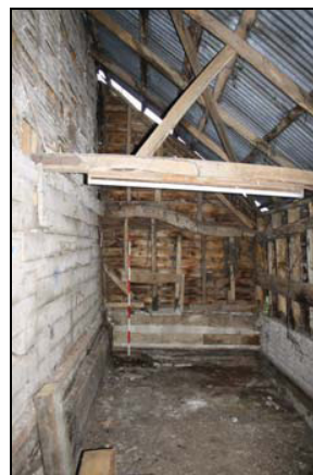
Curved bracing, porch interior, north-eastern elevation, taken from the south-west
