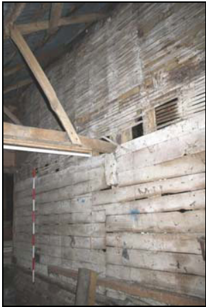
Upper laths and lower weather boarding, original external barn elevation seen in the outshut, taken from the north
