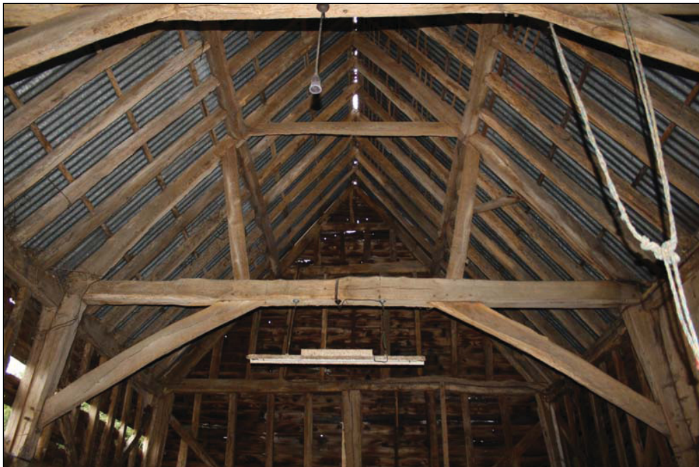
Plate 4 Truss and roof structure, taken from the north-west (DP 21)
