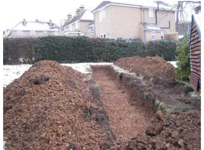
DP 8. SE part of the site with Trench 2. View WSW.
