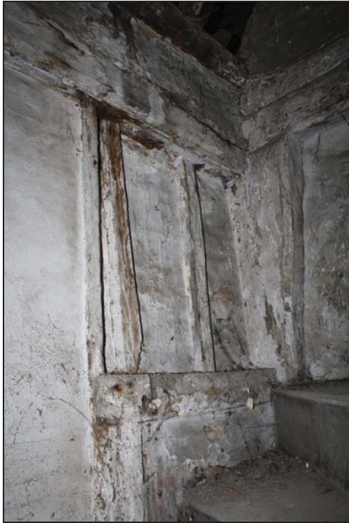
Detail of former window on the north wall of the old parlour chamber, now enclosed by the staircase, taken from the south-west
