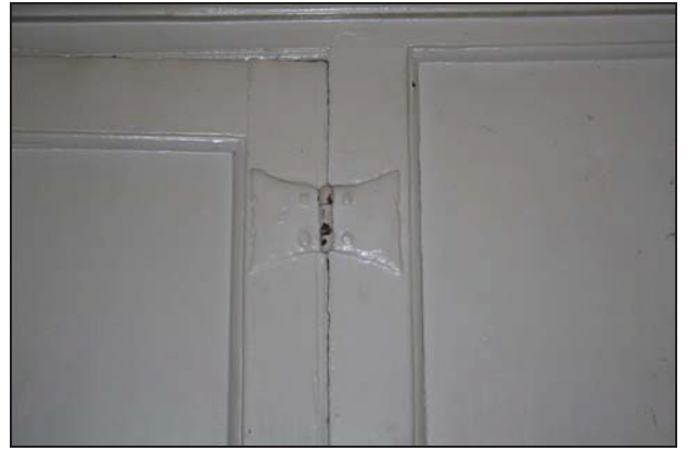
Butterfly-hinge on cupboard door in panelling on the north side of the hall chamber, taken from the south
