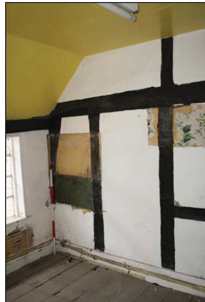
28 South side of the northern service chamber, taken from the north-west
