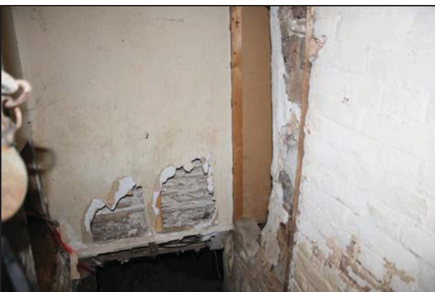
Detail on north side of the principal chimney stack showing lath and plasterwork behind modern lining, taken from the west
