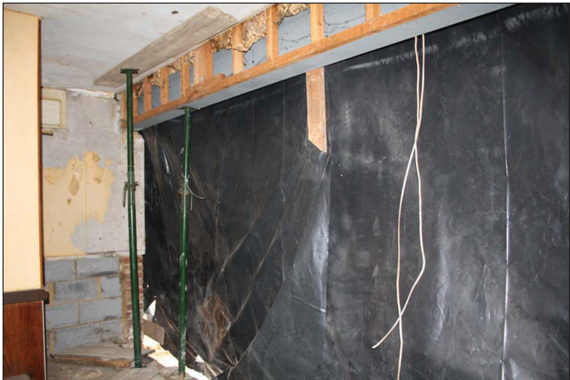
Plate 4 Detail of formerly external brickwork of the main range, taken from the south-west (5)
