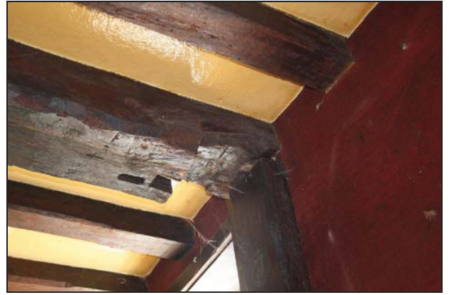
Binding joist on the south side of the hall showing evidence for the original jetty, taken from the north-west
