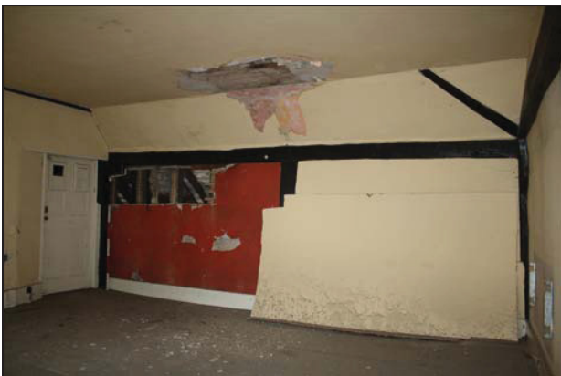
29 The second northern service chamber, taken from the south-east
