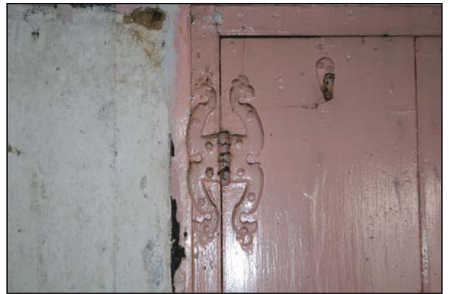
Detail of probably reused cockshead hinge on door to staircase on the north side of the parlour chamber, taken from the south
