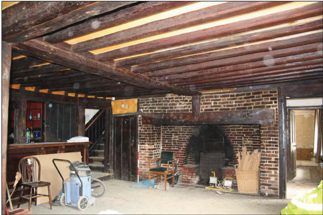
Plate 1 East side of the hall, taken from the west (09)
