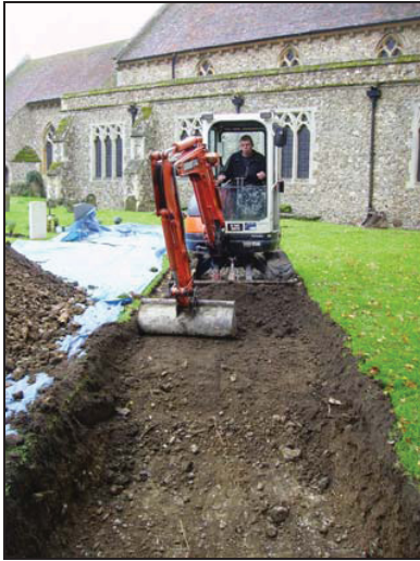
7 Excavating Trench 2. Looking southeast.
