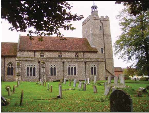
1 General view of the site. Looking south
