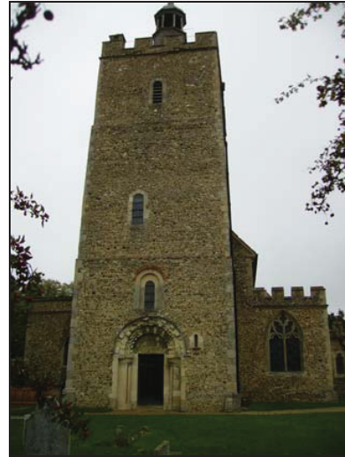
2 The 12 th century tower. Looking east.
