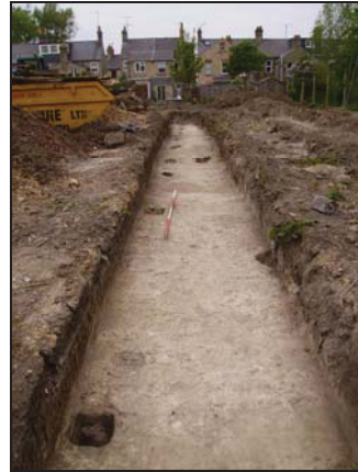
2 Trench 2. Excavated ditch with Ditton Walk properties in background. Looking north-west.
