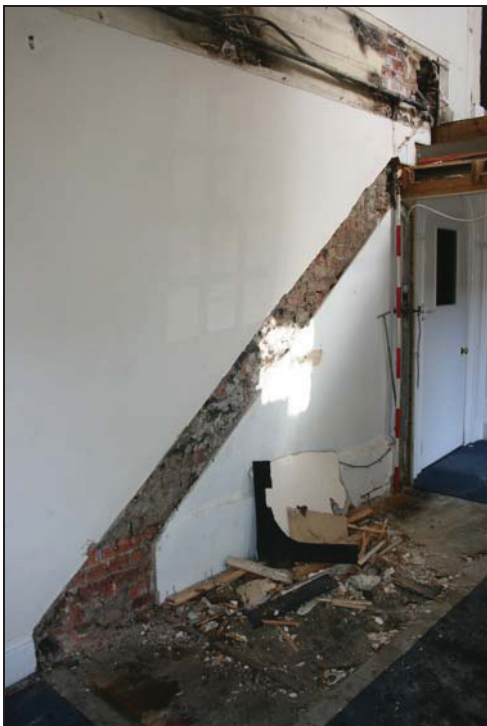
North-east side of the ground floor area showing exposed brickwork where staircase removed, taken from the west
