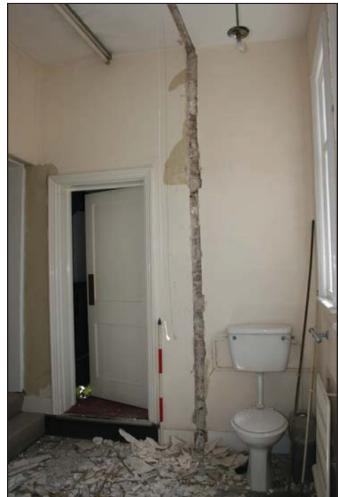
South-east wall of stair turret at first floor level showing removed partition, taken from the north-west
