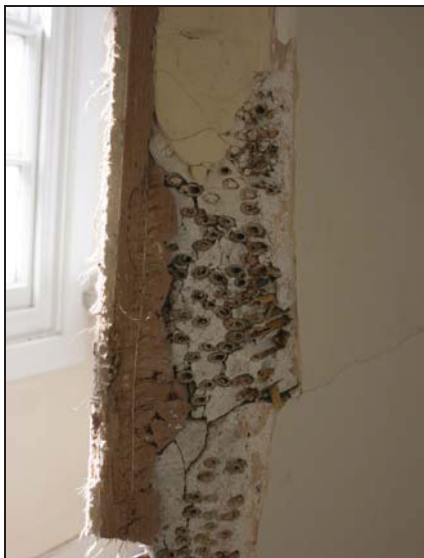
Detail of the fabric comprising the partitions at first floor level, taken from the east
