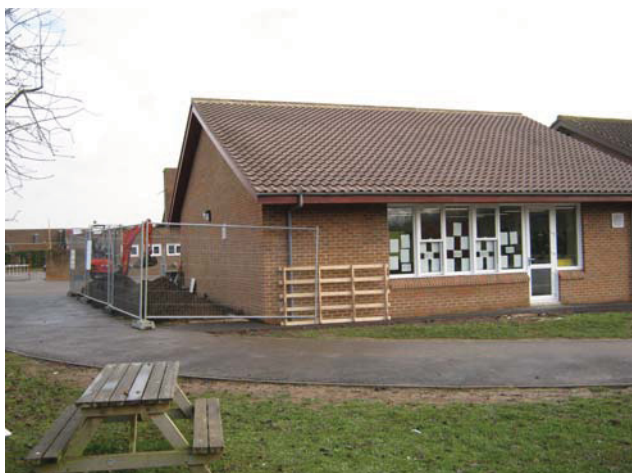
DP 1. Atwood Primary School, Sanderstead. New class room. View NE.
