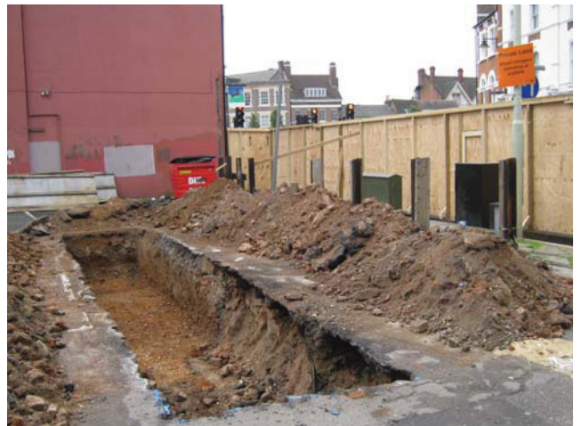
DP 6. Trench 2. View SSW.
