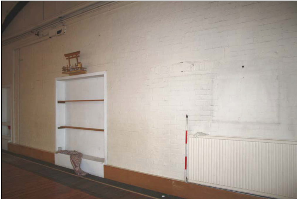
Plate 7 Blocked doorway and recessed cupboard, western elevation, taken from the north-east (DP 22)
