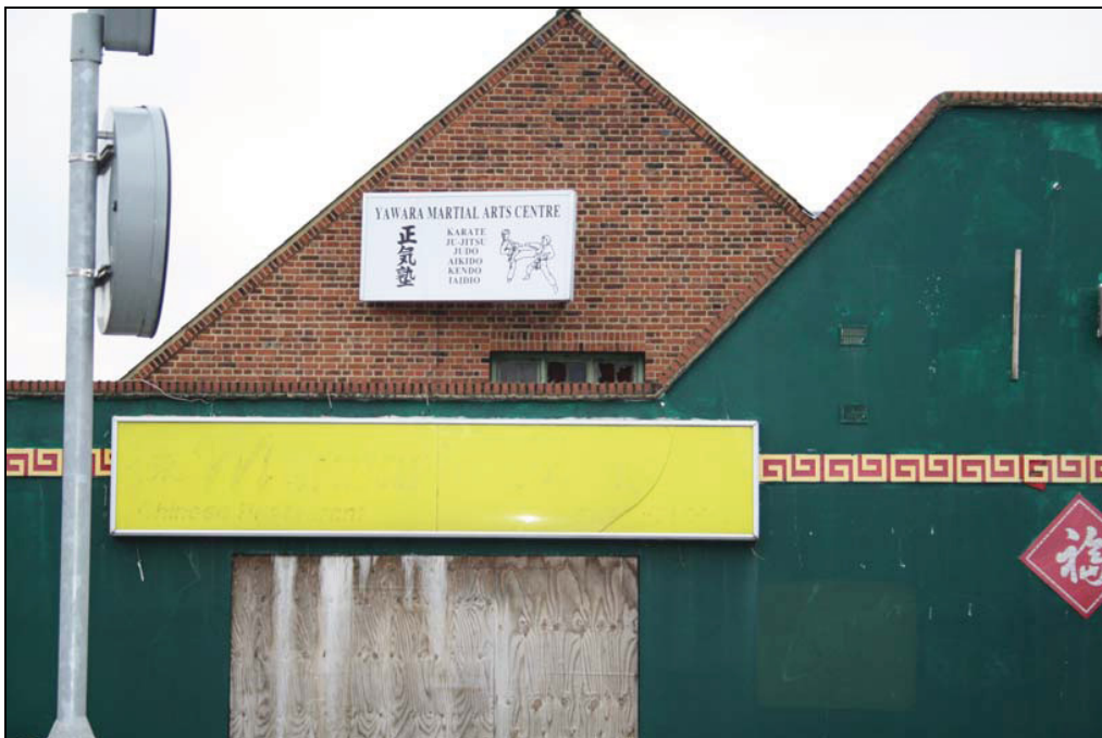
Plate 4 Blocked window at upper level, west elevation, yawara centre, taken from the west (DP 28)
