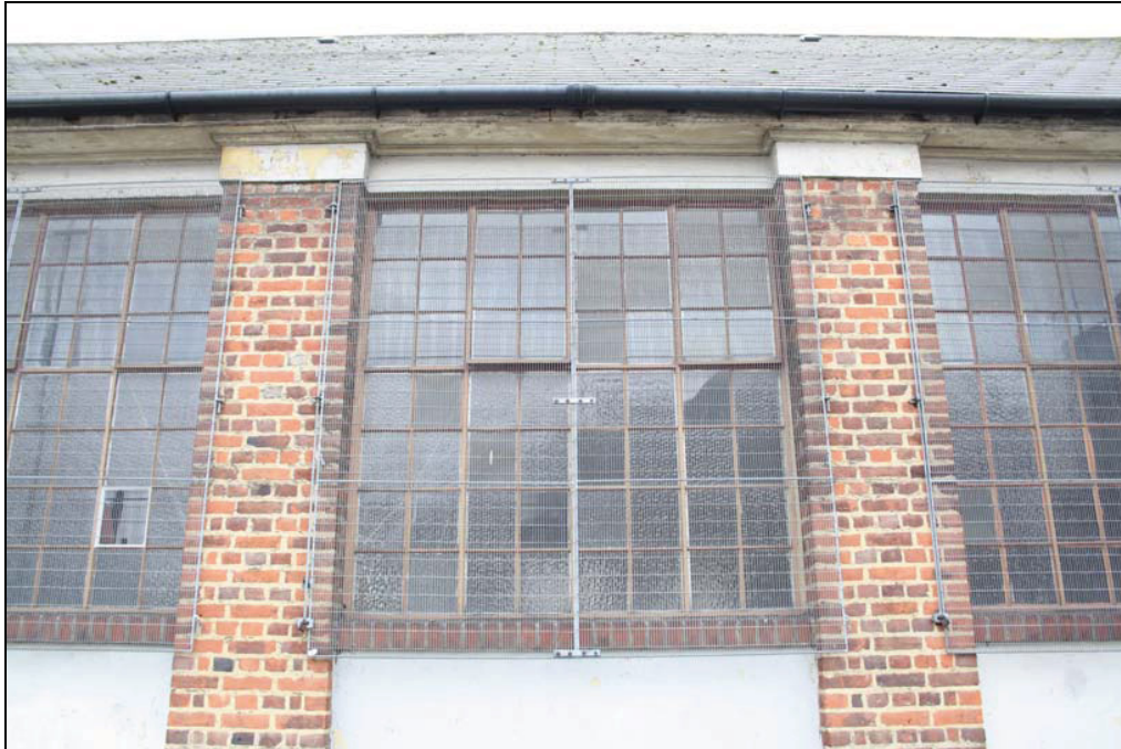
Plate 3 Original windows, northern elevation, taken from the north (DP 29)
