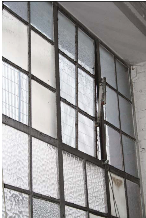
Plate 6 Pivoting upper casement, northern elevation, taken from the south-west (DP 24)
