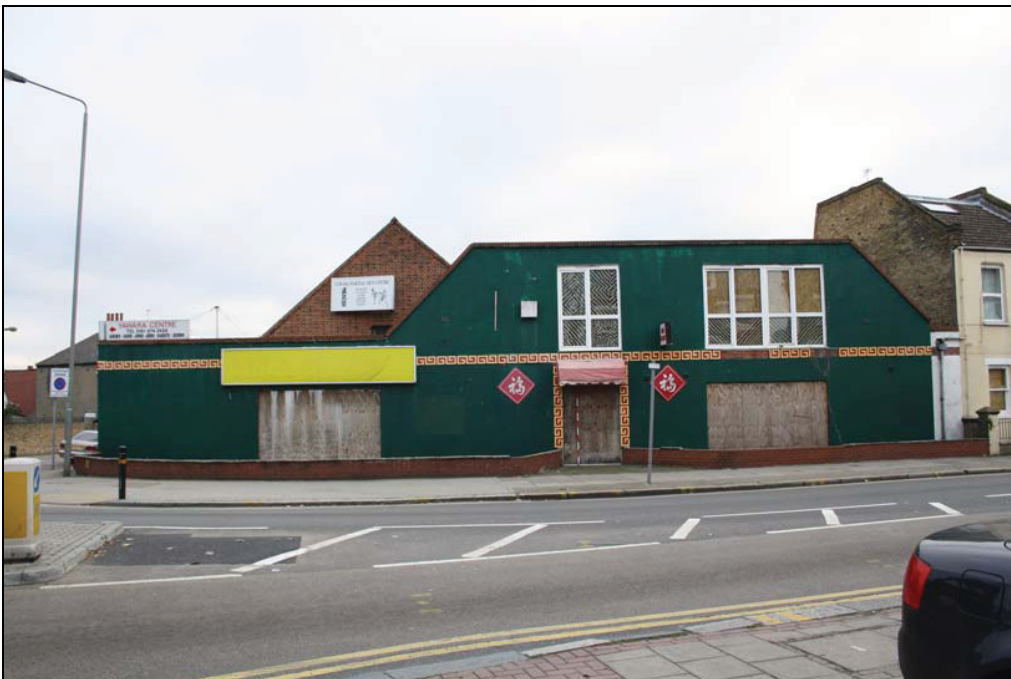
Plate 2 Yawara centre, taken from the west (DP 4)
