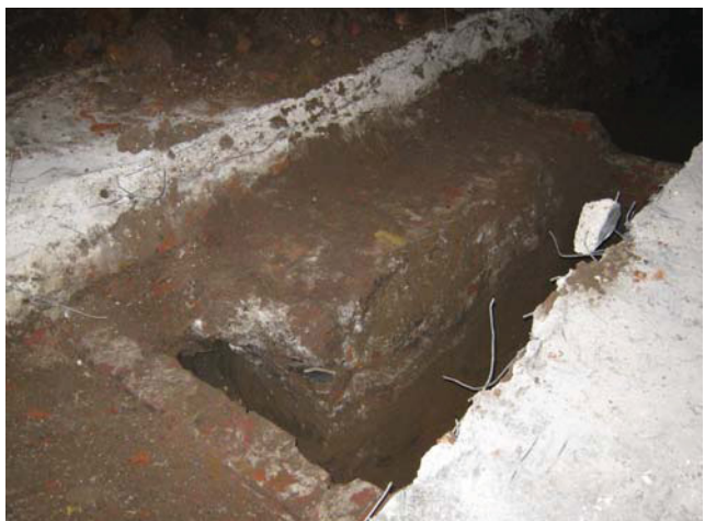
DP 18. Trench 2. Concrete ?slab M1008. View NW.
