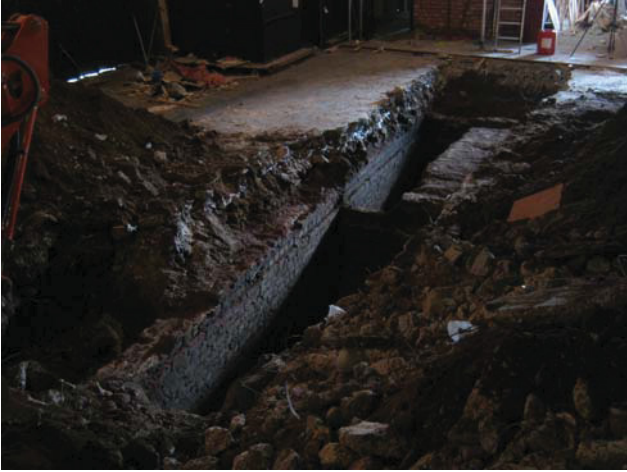
DP 13. Trench 2, Wall M1004. View SW.
