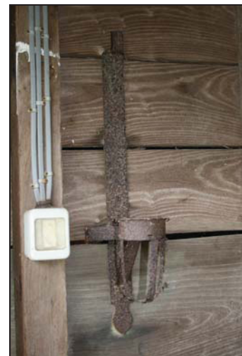
42 19 th century lamp holder on the western wall of Bay 13, taken from the south-west
