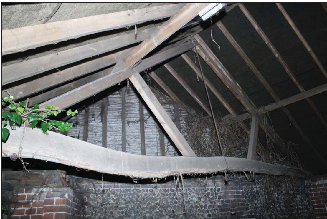
Plate 8 Bay 14, roof truss, taken from the west (20)
