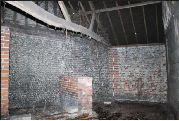
19 Bay 14 with internal brick partitions, taken from the north-west
