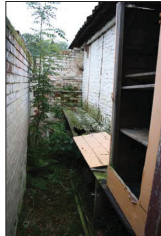
40 The remains of shelving within the potting shed, taken from the north-east
