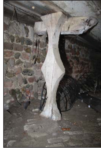
38 Shaped support for work tops in potting shed, taken from the south-west
