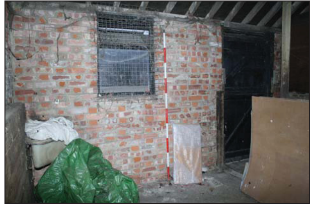
Stable door and window showing Fletton brick inner face of Bay 9, taken from the south-east
