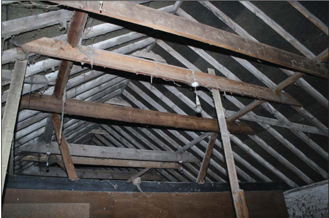
5 Roof structure above Bays 10 and 9, taken from the south-west (26)
