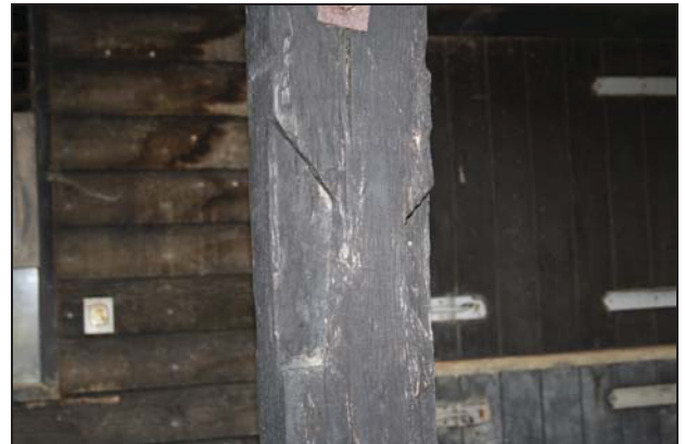
34 Supporting post between Bays 7 and 8, retaining redundant mortices, taken from the north-west
