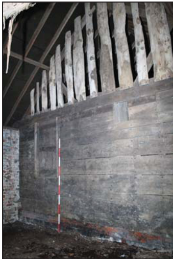
21 Partition between Bays 14 and 13, taken from the north
