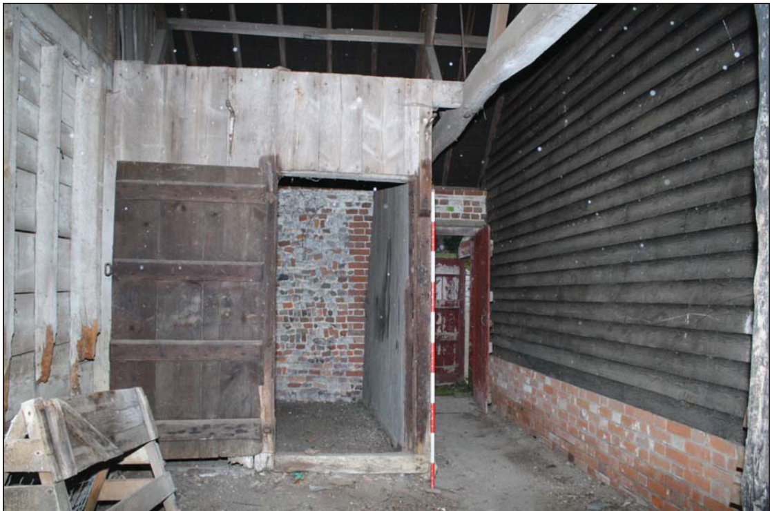
6 Bay 13, internal pen, taken from the north-west (22)
