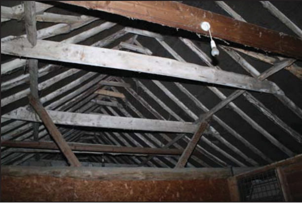
31 Roof structure above Bays 7 & 8, taken from the east
