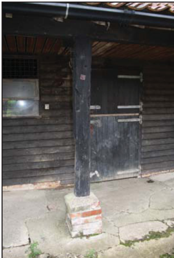
35 Supporting post on brick stylobate between Bays 6 and 7, taken from the north-west
