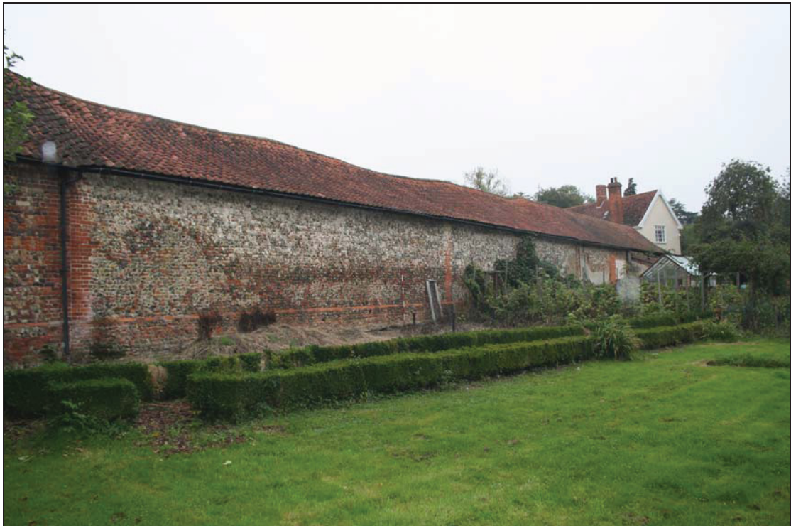
1 South-east elevation, taken from the south (14)
