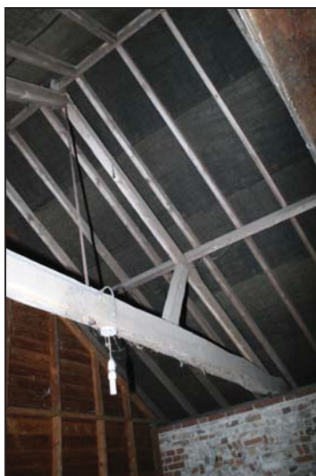
23 Roof truss, Bay 12, taken from the north-west
