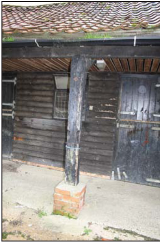
33 Supporting post on brick stylobate between Bays 7 & 8, taken from the north
