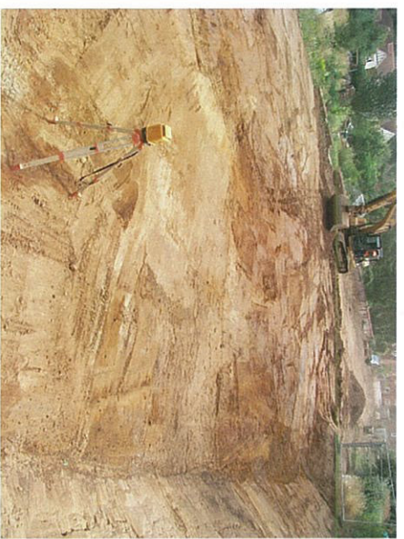
DP4. Garden terracing, looking SE.
