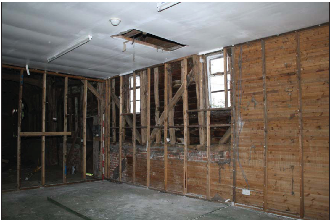
6 Bays 6 & 7, western wall panels, taken from the north (17)
