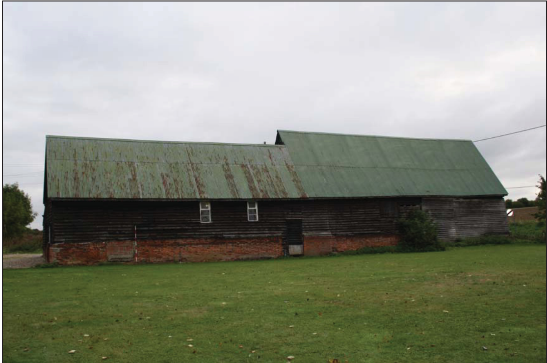
1 South-west elevation of the barn, taken from the south-west (01)
