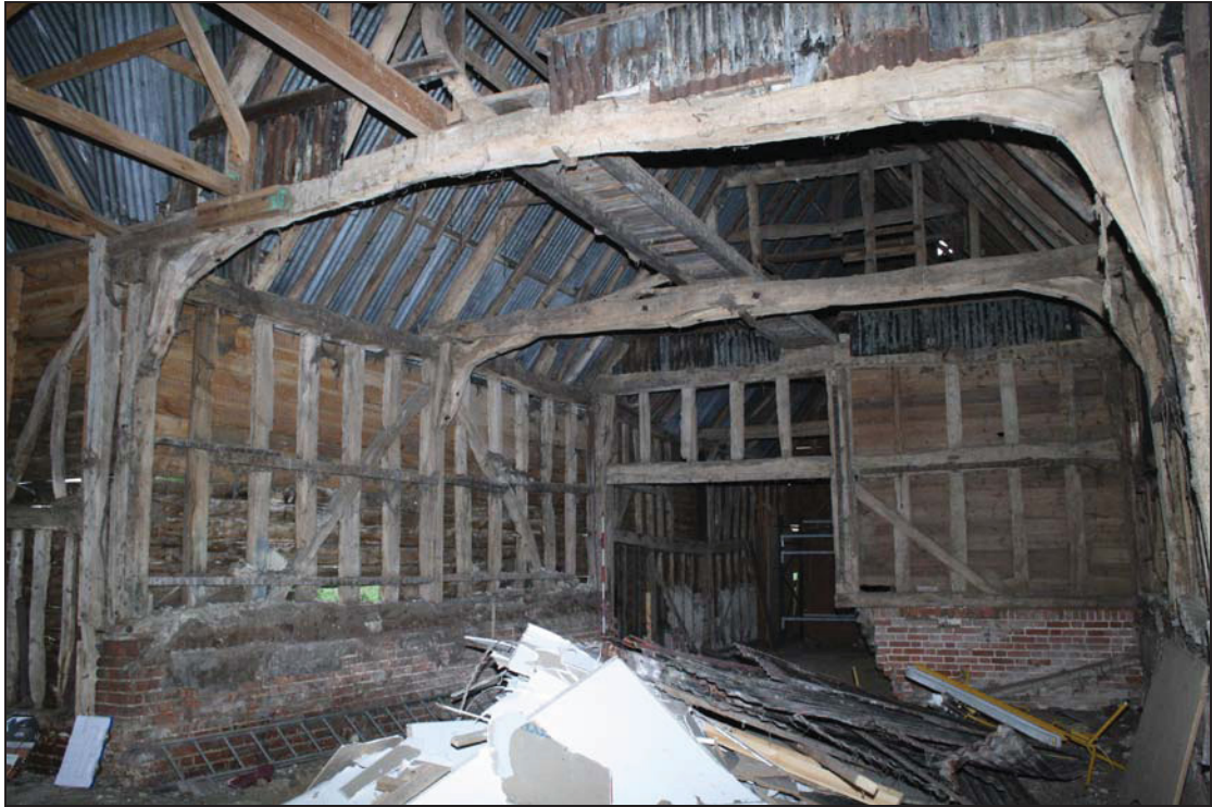
3 Bays 3 & 4, taken from the north-west (10)
