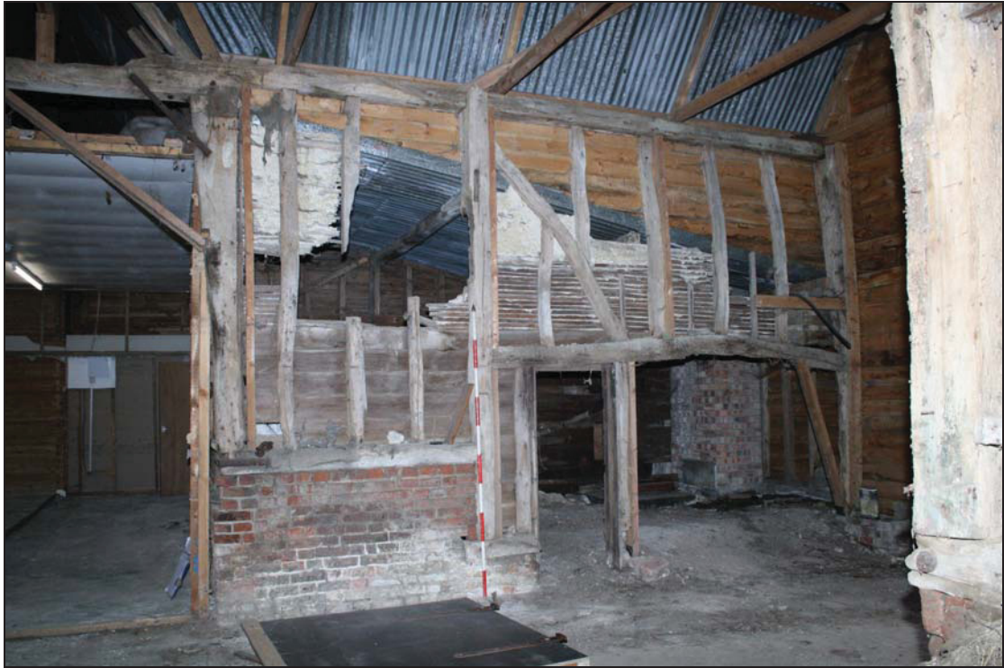
5 Midstrete (Bay 5), north-west wall panel, taken from the south (14)
