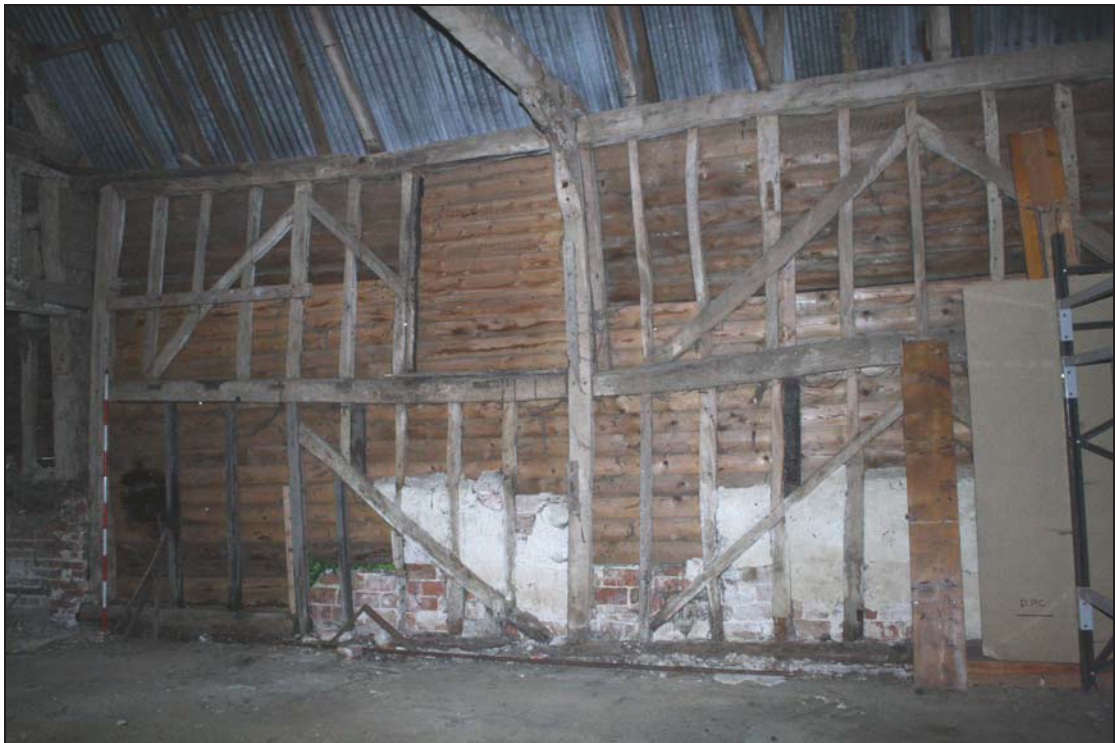
Plate 8 Bays 1 & 2, eastern wall panels, taken from the south-west (07)
