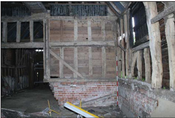
Former tie-beam, reused as the west post of Bay 2, taken from the south-east
