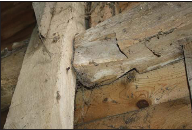
Former tie-beam reused as a mid-rail on the north-east wall of Bay 1, taken from the south
