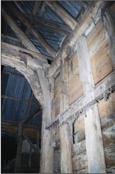
Redundant notch lap joints for a brace, north-east side of Bay 4, taken from the south
