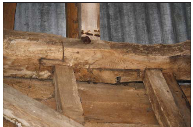
Face-halved and bladed scarf joint in the wall-plate of Bay 2 (north-east side), taken from the west
