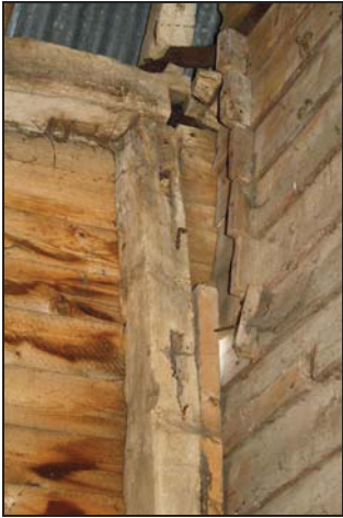
Former tie-beam, reused as the west post of Bay 2, taken from the south-east
