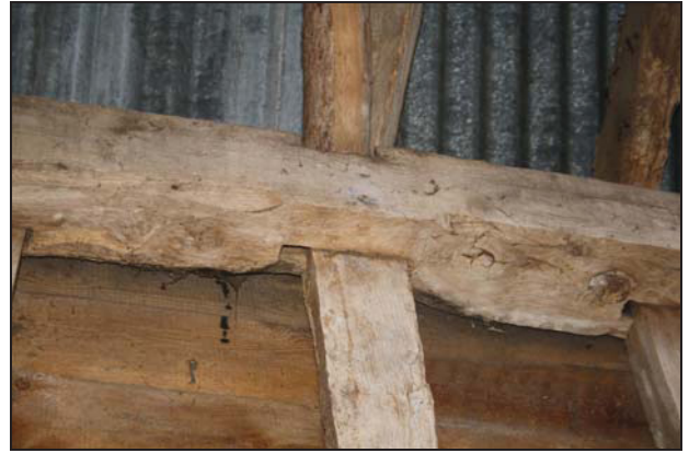
Unused configuration for a bay division post, positioned to the south of the actual bay division on the north-east wall of Bay 1, taken from the west
