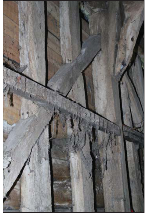
Original tension brace, in situ, north-east side of Bay 4, taken from the west
