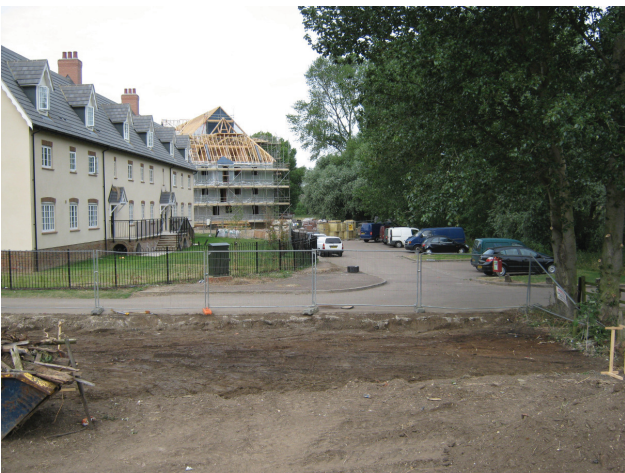
DP 3. The site. View W.
