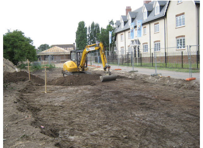
DP 2. Ground reduction in progress. View SSW.
