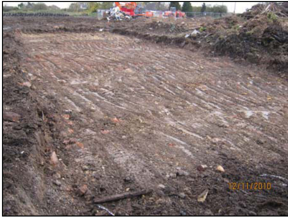
1 Footprint of Building 9. Looking north-west
