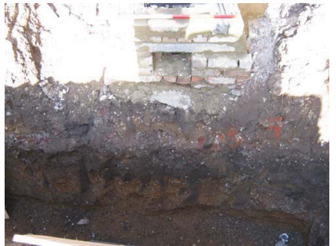
DP 6. W foundation trench. Sample section. View W.
