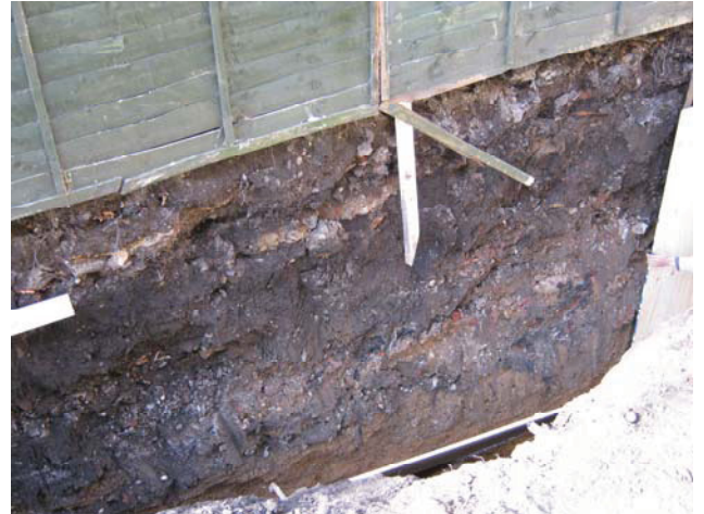
DP 8. S foundation trench. View SSW.
