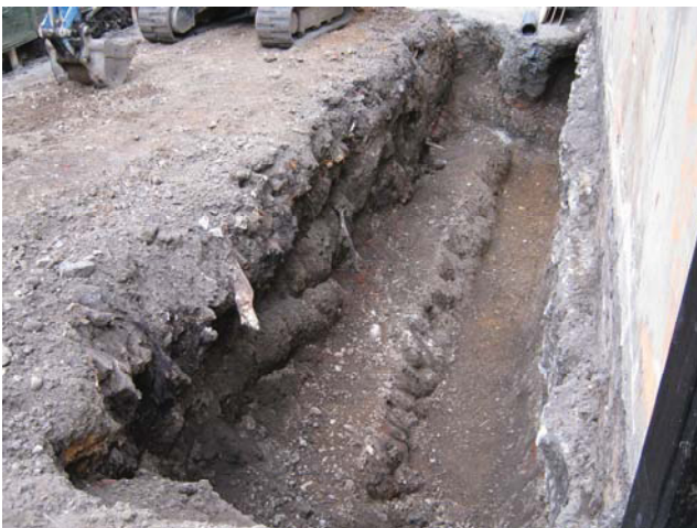
DP 5. N foundation trench. View W.
