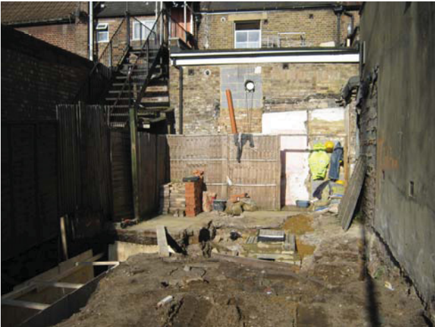
DP 3. The site. View W.
