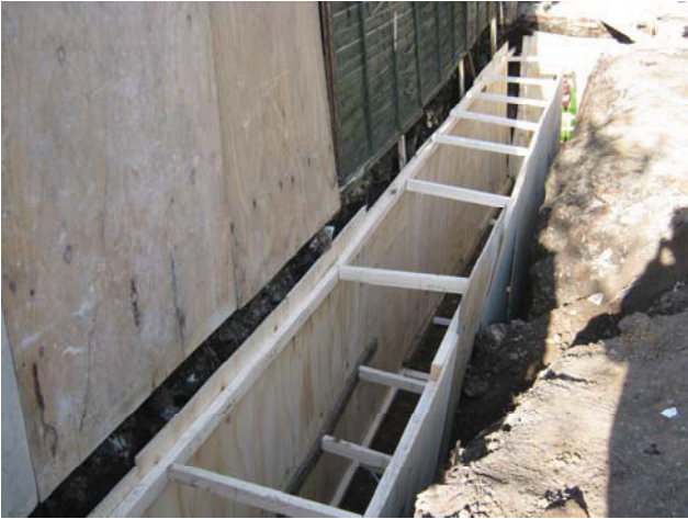
DP 7. S foundation trench. View WSW.
