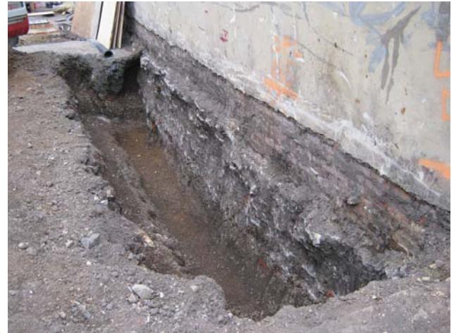
DP 4. N foundation trench. View WNW.
