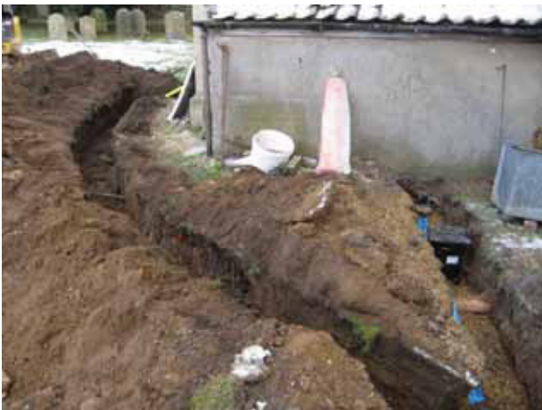
15 Post-excitation view of trenches north side of the nave. Looking east.
