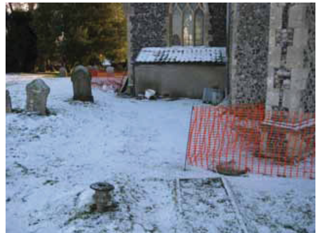
16 View of backfilled trenches north side of the nave. Looking east.
