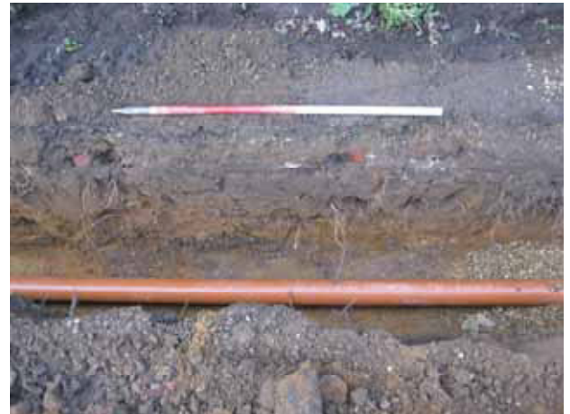
14 Sample section 4. Looking west.
