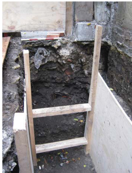
DP 4. S foundation trench, E end. View E.
