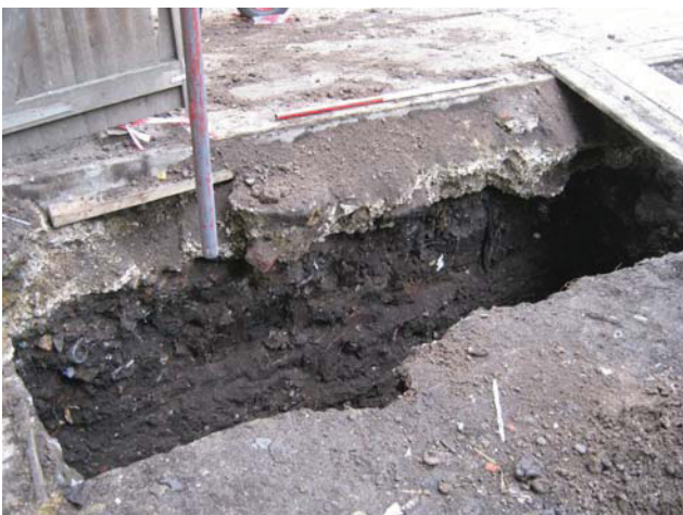
DP 5. E foundation trench. View SE.
