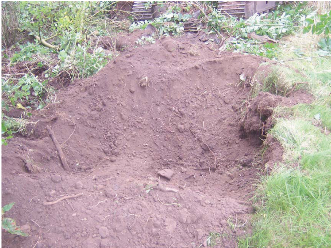
Plate 2 Removal of trees in topsoil (1001) looking south-east.
