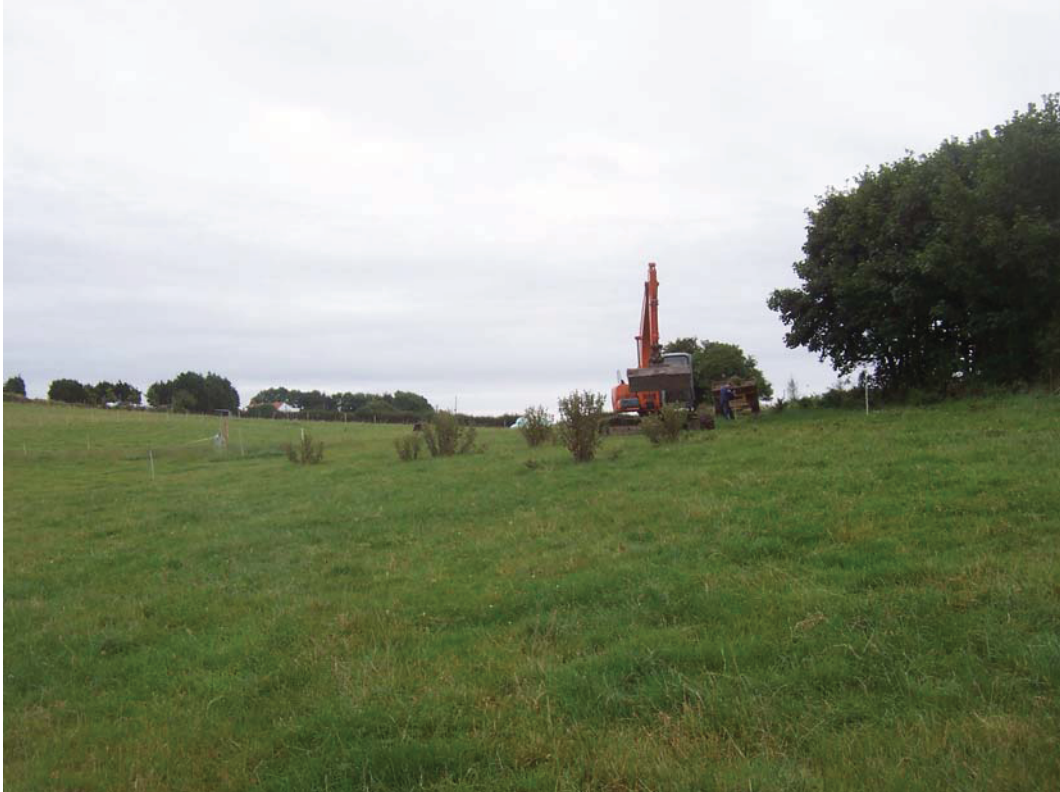
Plate 3 The application area proper, note the lie of the land, dropping sharply to the east necessitating the build up of ground rather than any stripping, viewed from the north.
