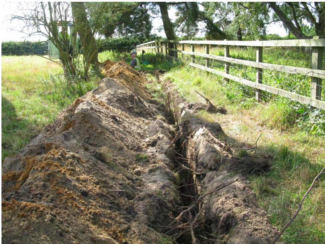
Plate 4 Trench 1 looking south through the wooded area to Top Road.
