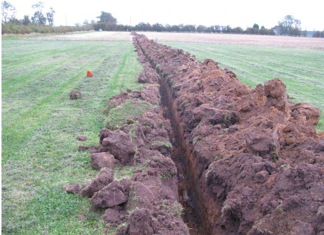
Plate 19 Trench 10, looking east.
