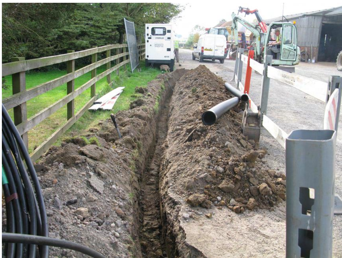
Plate 22 Trench 11 during excavation in the farm yard.
