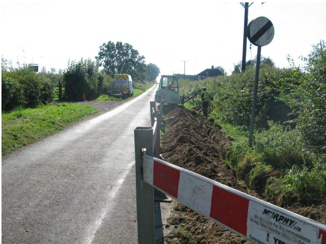
Plate 18 Trench 9 on the west side of Mill Lane, looking south.
