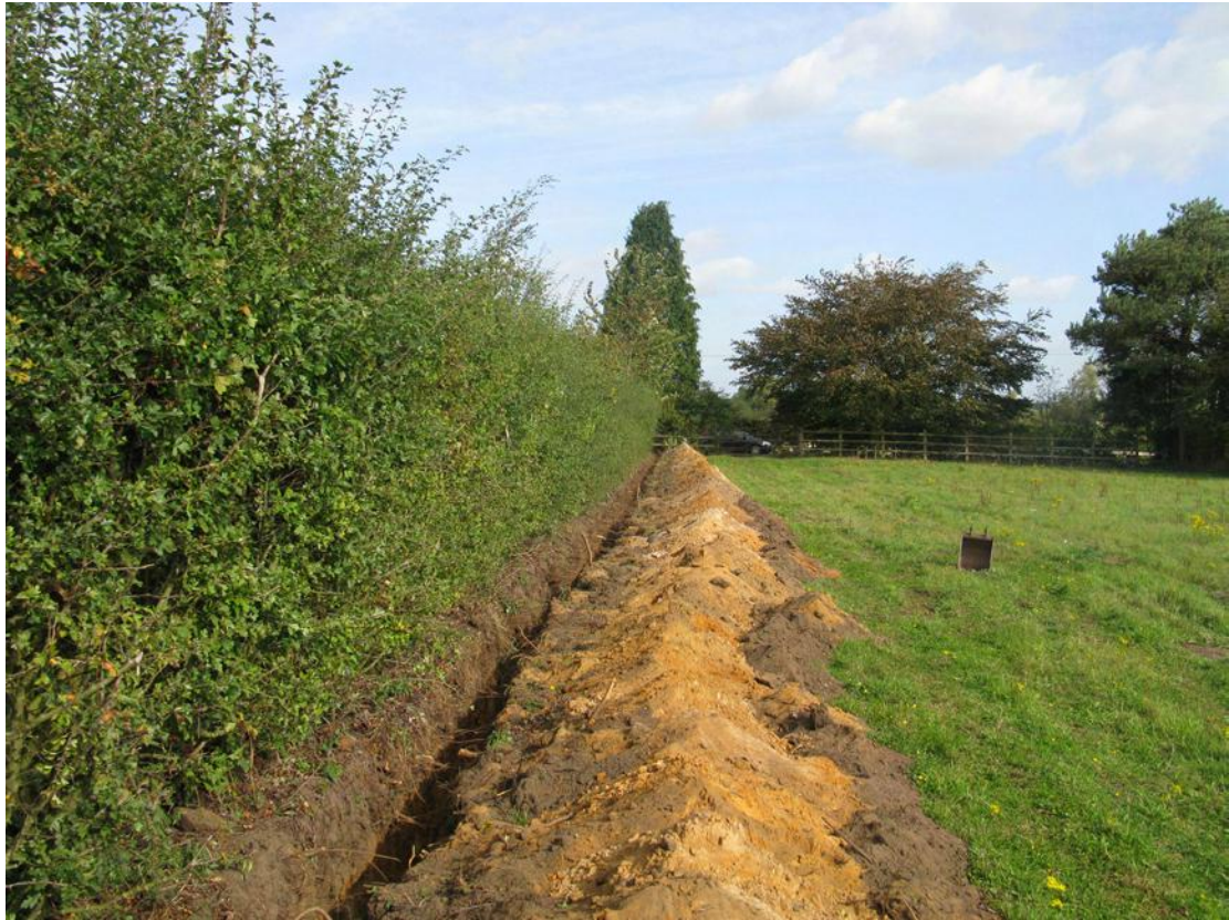
Plate 15 Trench 8, looking north to Low Road.
