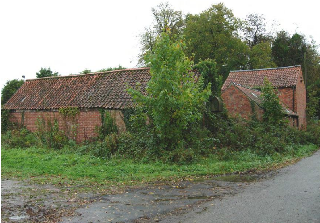
Plate 1 General view of the site from the south-west
