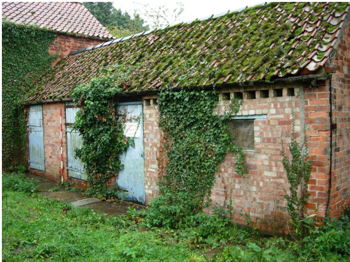
Plate 6 North elevation of building B
