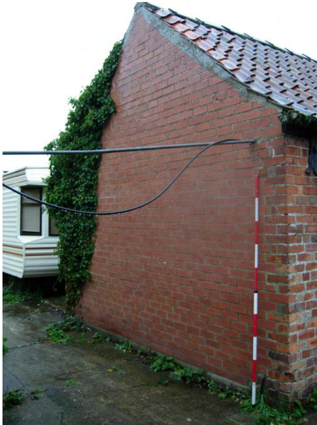
Plate 11 West elevation of building C
