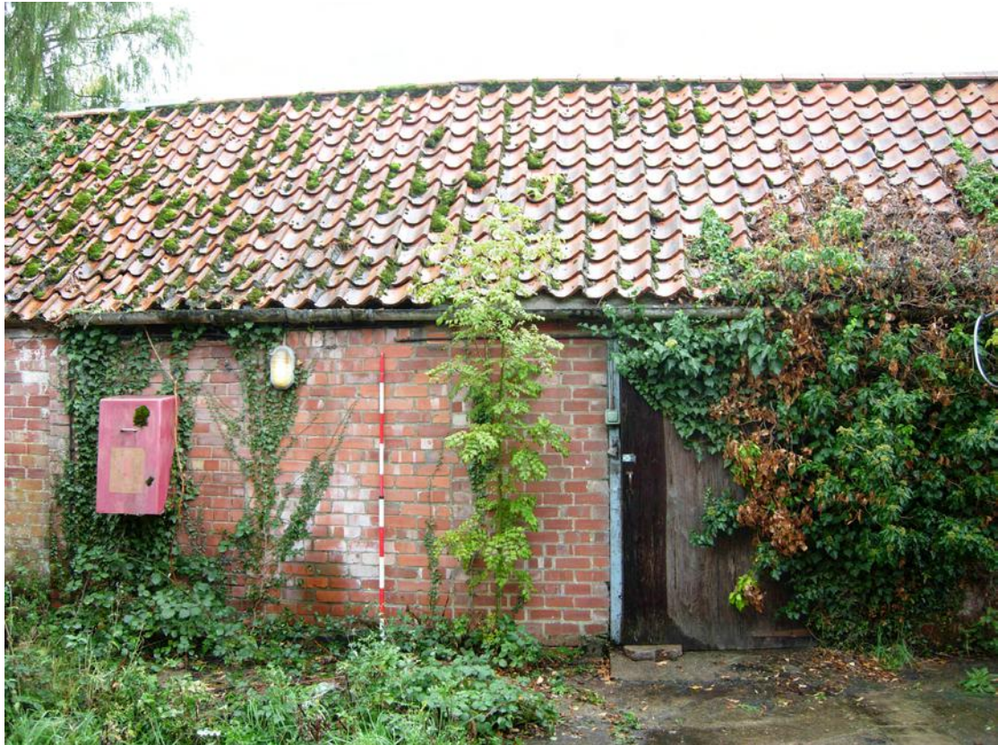
Plate 15 Central portion of the east elevation of building D
