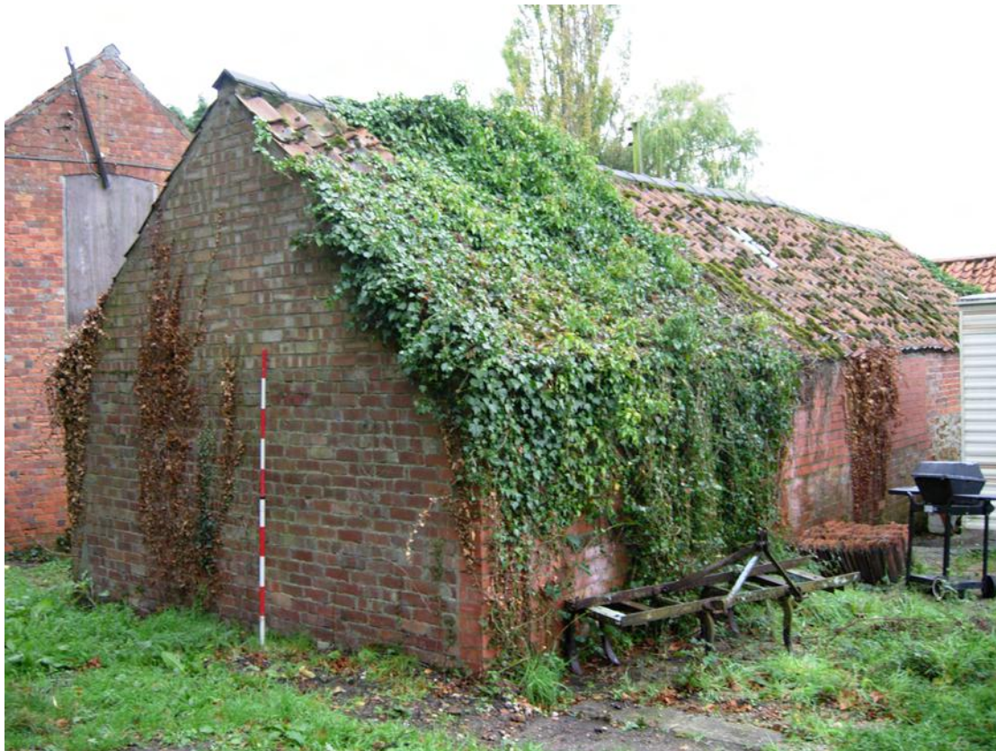
Plate 12 East elevation and part of the north elevation of building C
