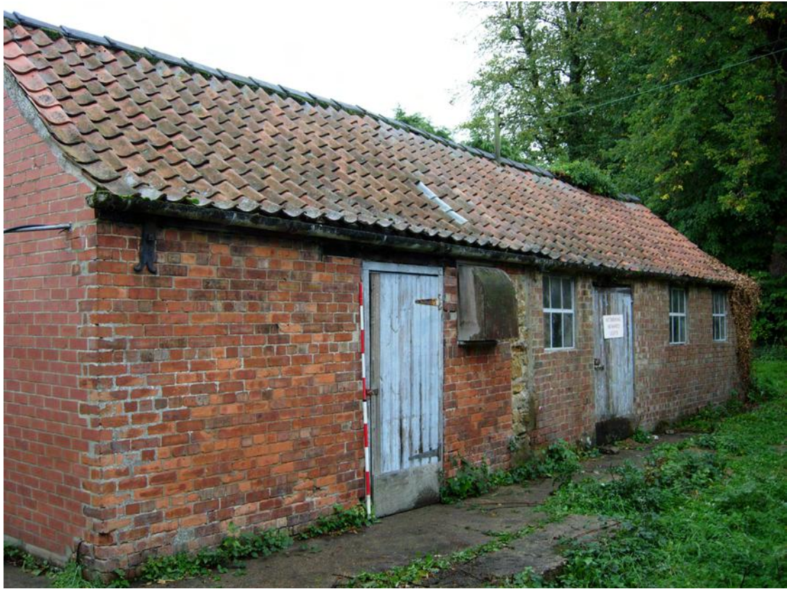
Plate 9 South elevation of building C
