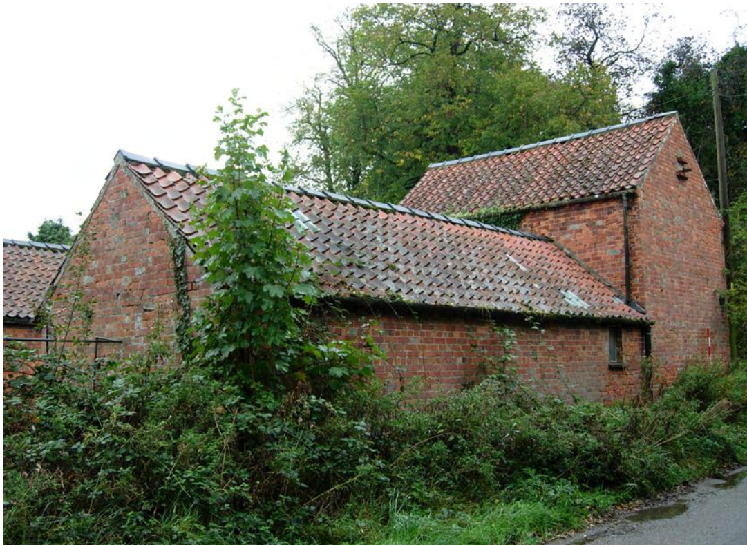
Plate 8 South and west elevations of building B with building A in the background
