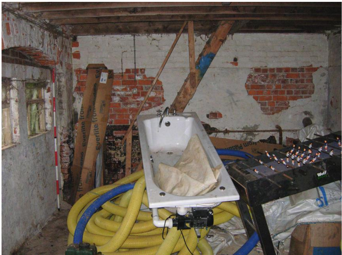
Plate 18 Ground floor of building A, looking south
