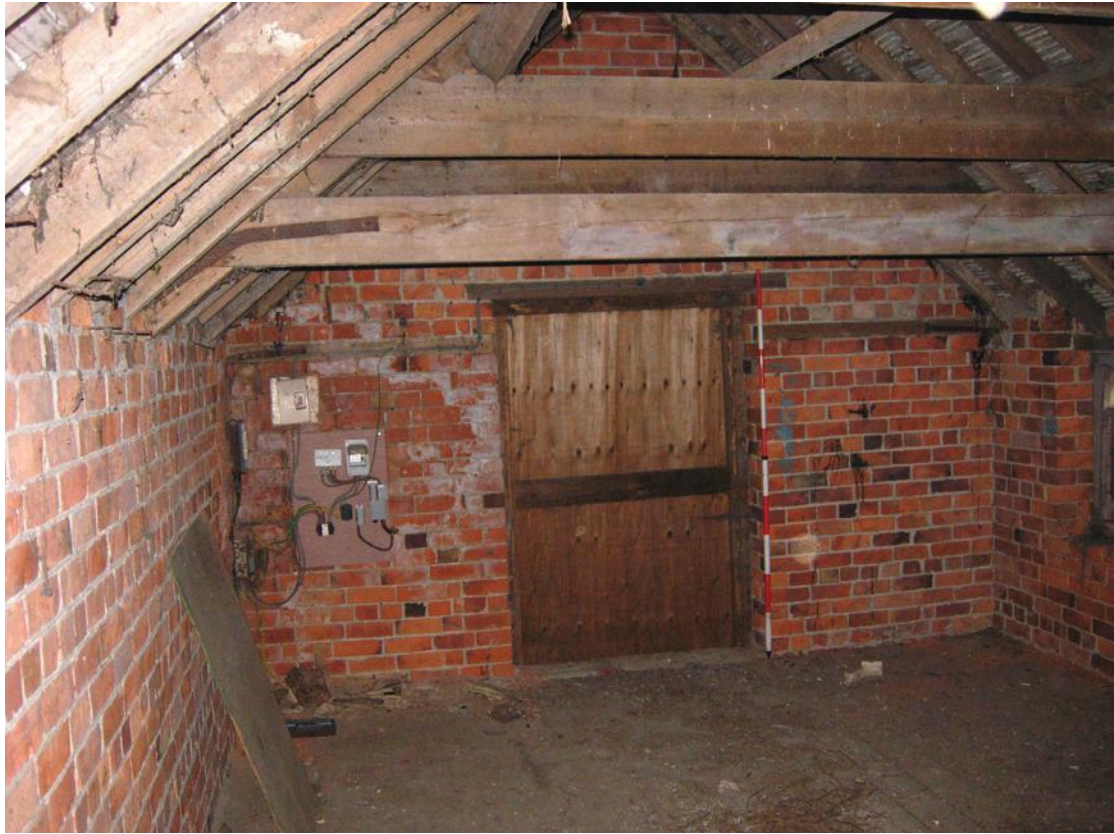
Plate 19 First floor of building A, looking north
